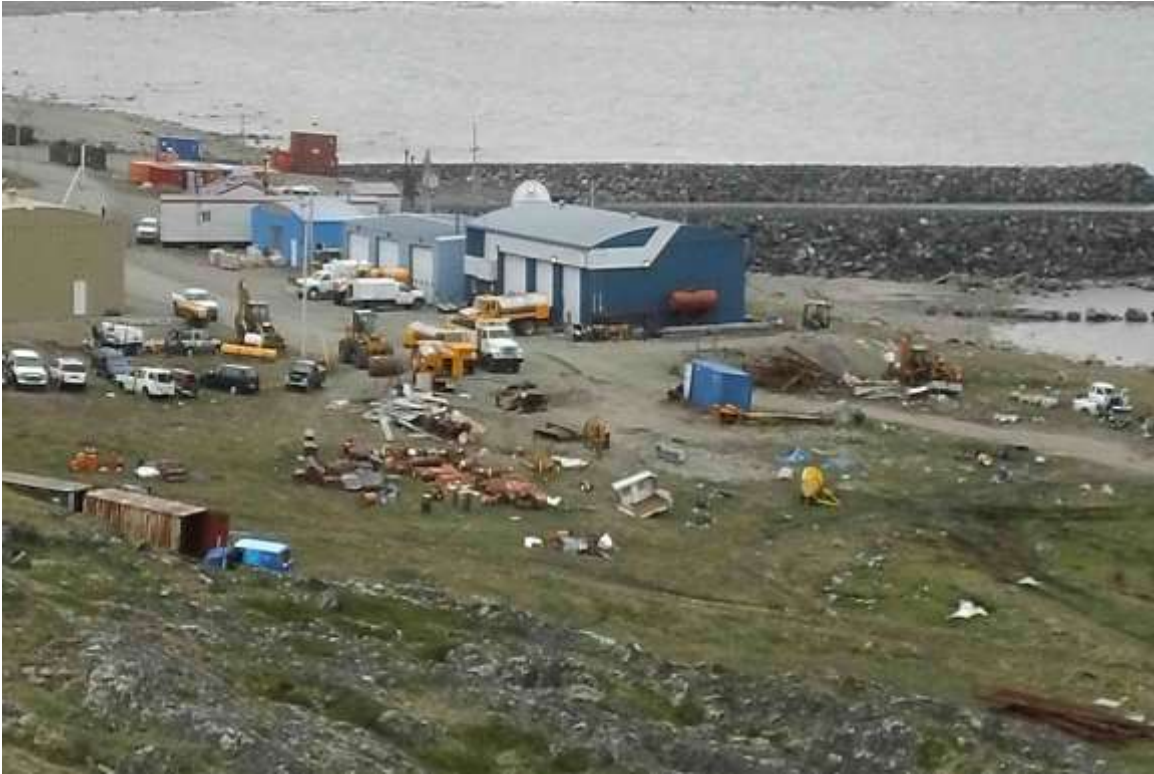
Figure 8: View of municipal garage area after material was removed, August 2013
