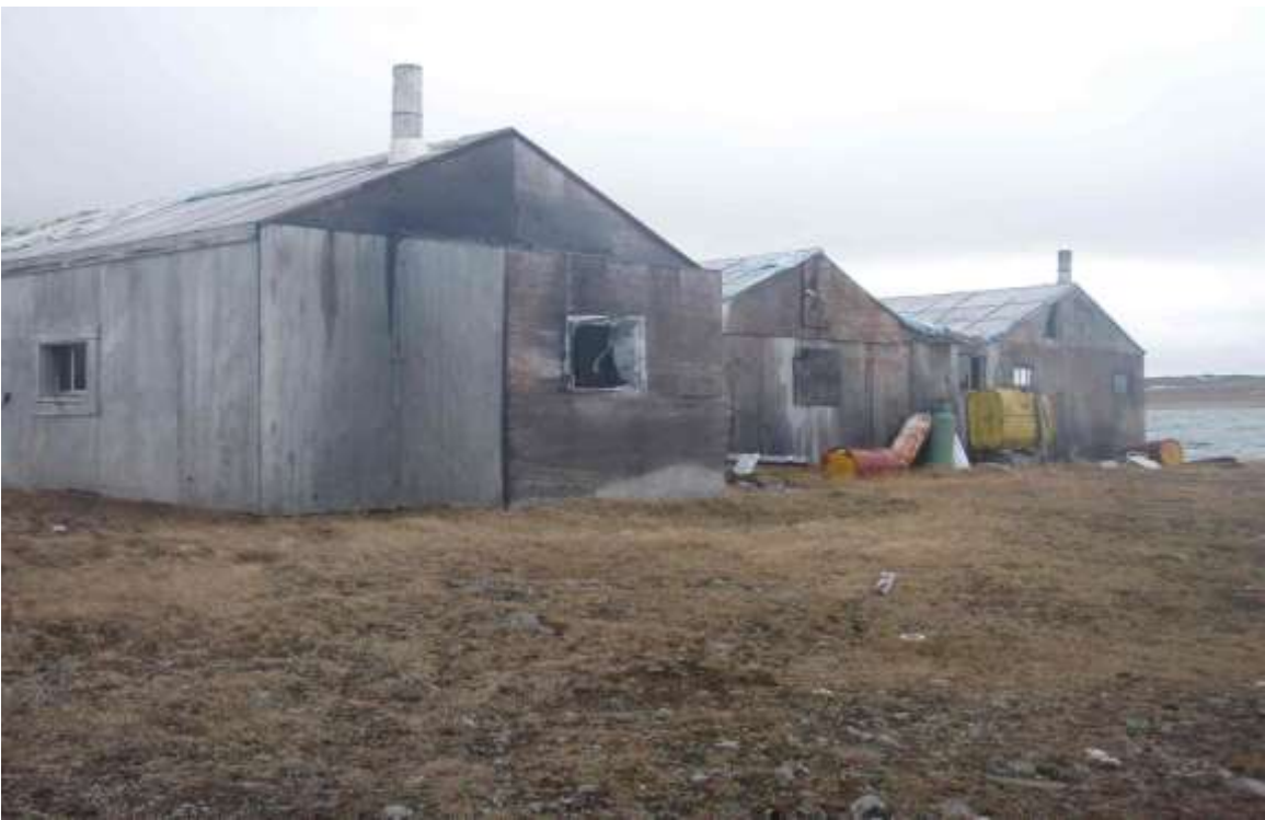
Figure 26: Example of wooden structures and debris found on site WB-9, June 2012
