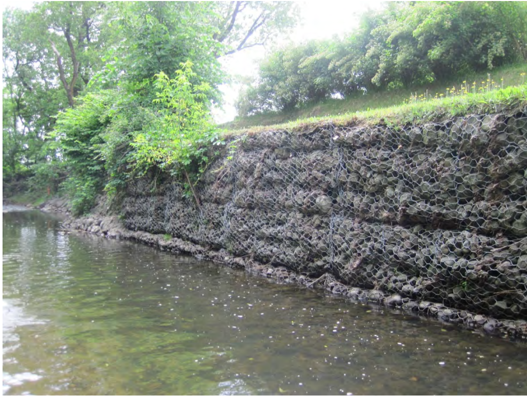
Figure 3.19 Mur de gabions
