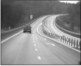
Source : National Road Authority, Irlande, 2004
