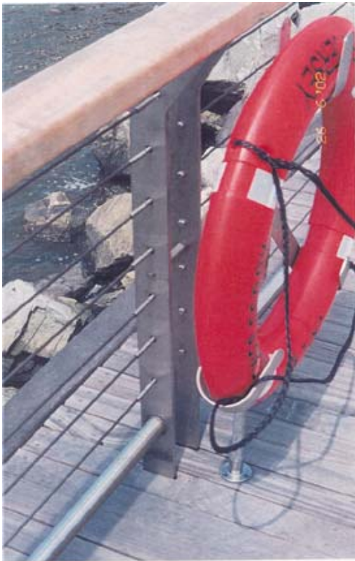
Photo #23 Garde-corps, Cape May, N.J.
