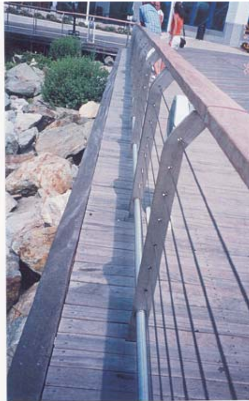
Photo #24 Garde-corps, Cape May, N.J.
