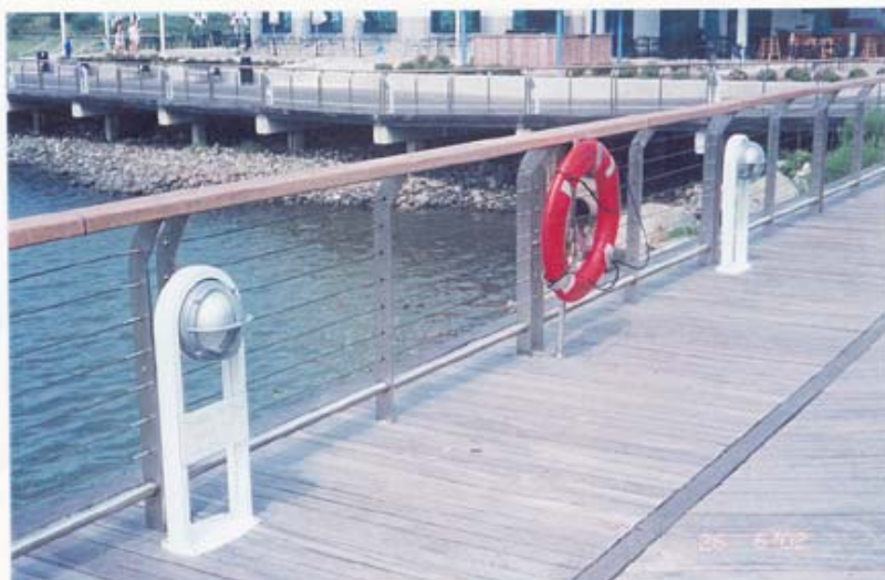
Photo #25 Garde-corps, Cape May, N.J.
