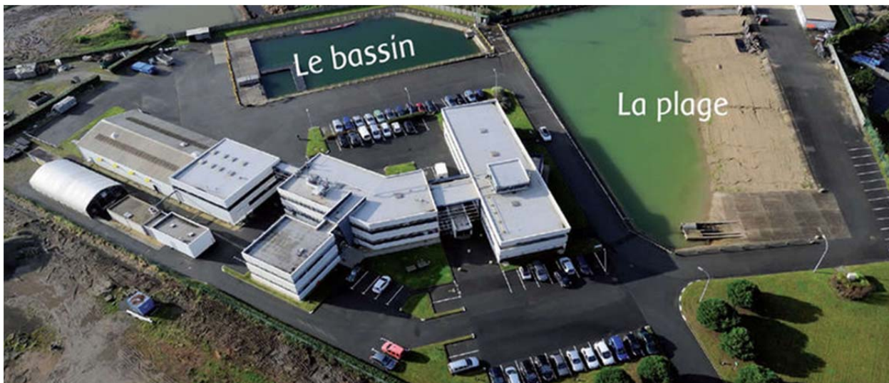
Figure 17 Installations du CEDRE
