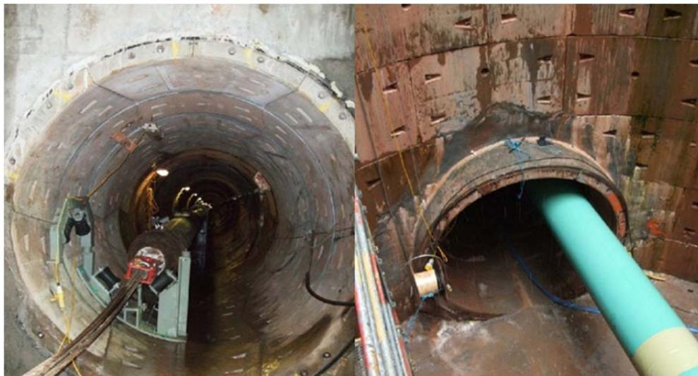
**FIGURE 6-7 – INSTALLATION DES TUYAUX DANS LE TUNNEL SOUS LA RIVIÈRE EXE (SOURCE – SITE INTERNET DE *BDGSMITH ENGINEERING EXPATRIATES*).**
