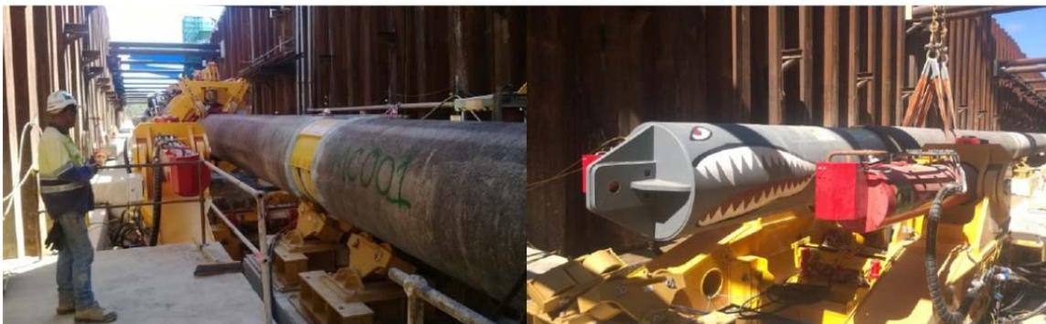
**FIGURE 6-10 – EXEMPLE DE "PIPE THRUSTER" INSTALLANT UN PIPELINE AVEC REVÈTEMENT EN BETON DANS UN TUNNEL EXISTANT TUNNEL EN AUSTRALIE (PFEFF, 2014).**
