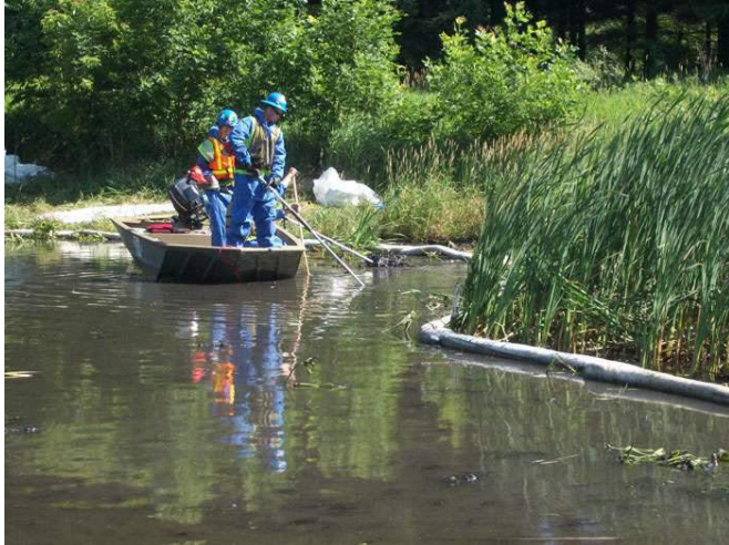
Figure 8.11 Agitation of Kalamazoo River sediment with jets of water to flush submerged oil to the surface. Image from US EPA.
