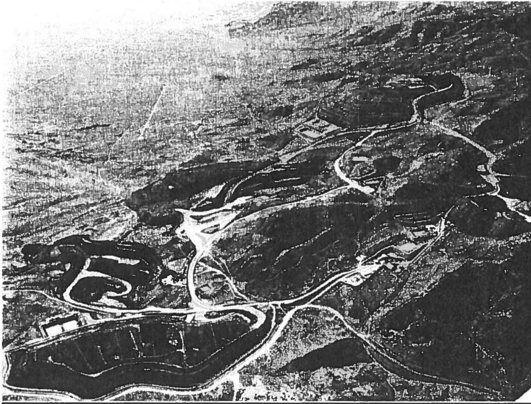
Figure 7a. The Rand Mine located near Randsburg, California. Two open pits are evident, along with a cyanide leach pad in the lower right, and two large waste piles in the central portion of the image. The larger cyanide leach pad in the upper right of the image is about 1.8 by 2.1 miles in extent.
