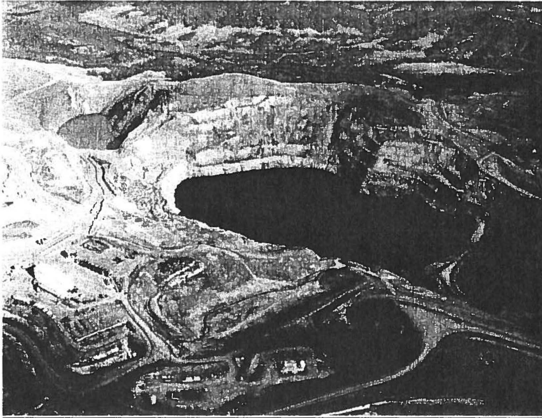
Figure 2. Homestake's McLaughlin Mine in northern California. The main pit is approximately a mile in length and 750 feet deep, with acid water. The smaller pit is also considered reclaimed.
