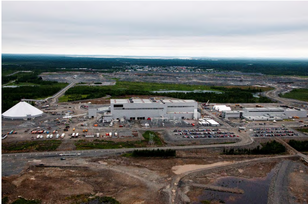
Figure 18.1 – Aerial view of the infrastructure of the Canadian Malartic mine (looking north)
