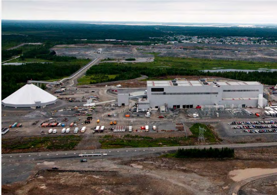
Figure 17.2 – Aerial view of the process facilities
