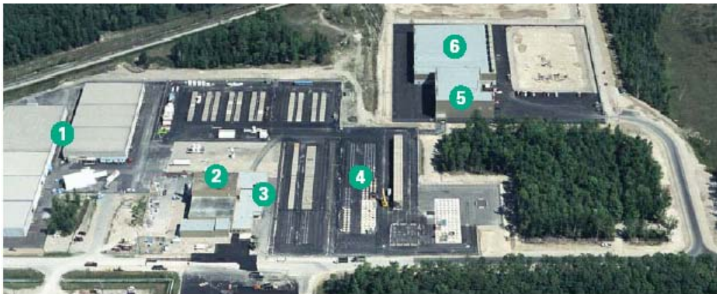
Aerial view of Ontario Power Generation's Western Waste Management Facility (WWMF), showing 1. Low Level Storage Buildings, 2. Waste Volume Reduction Building, 3. Amenities Building, 4. In-ground containers, 5. Western Used Fuel Dry Storage Facility Processing Building, and 6. Dry Storage Container (DSC) Storage Building.
