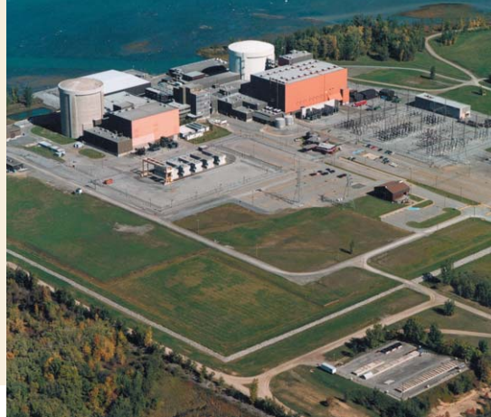
Aerial view of Gentilly nuclear complex
