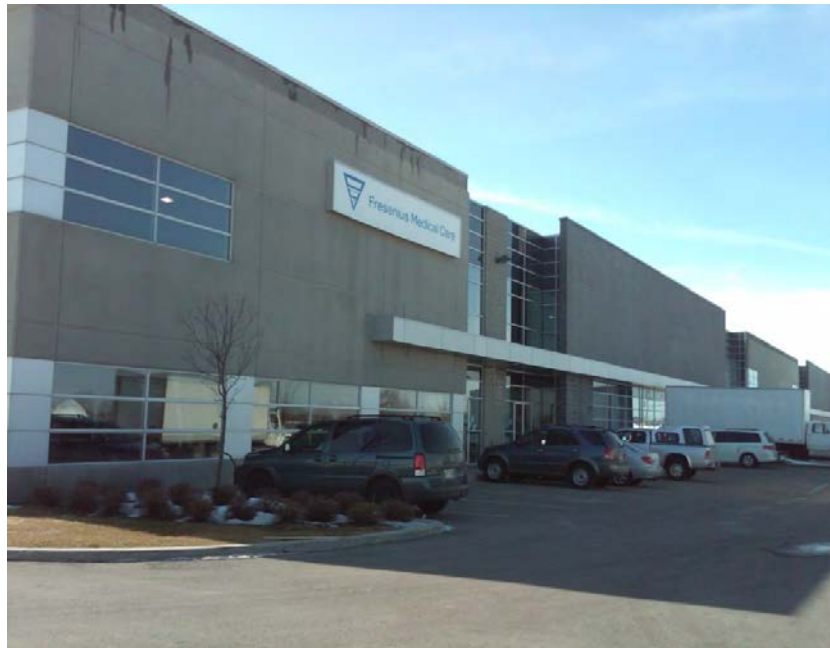
Figure 1: General view of the building located at 3600 F.X. Tessier Street. View toward the south.
