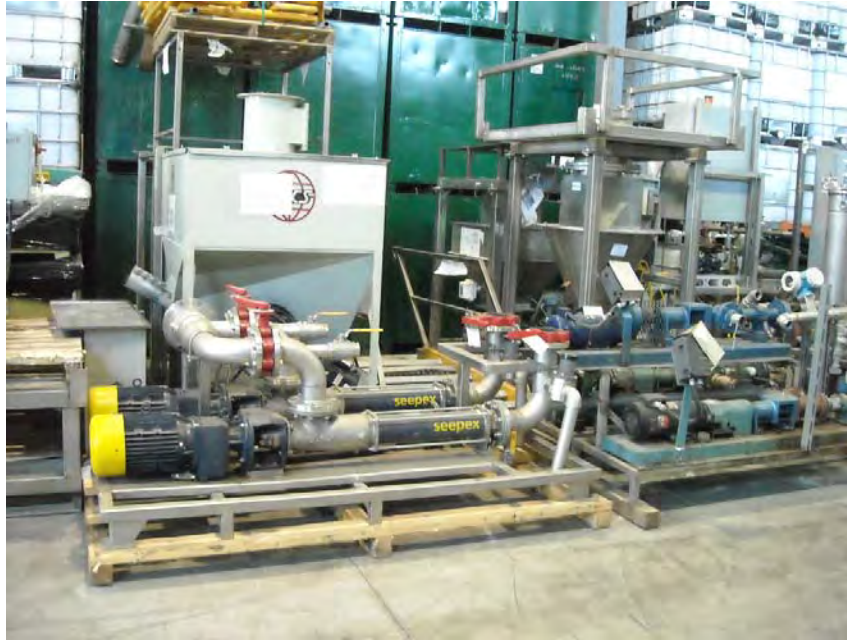
Figure 3: General view of the storage observed inside the suite occupied by Buckman Laboratories of Canada (3600 F.X. Tessier Street).
