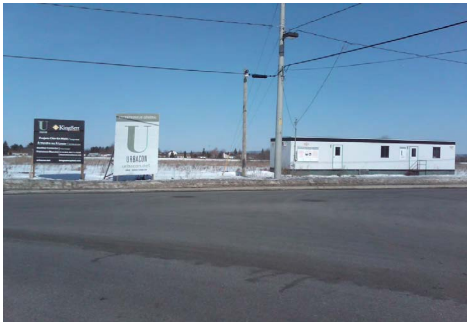
Figure 22: Partial view of a field trailer observed in the portion of the Site consisting of vacant lots located on the north side of F.X. Tessier Street.
