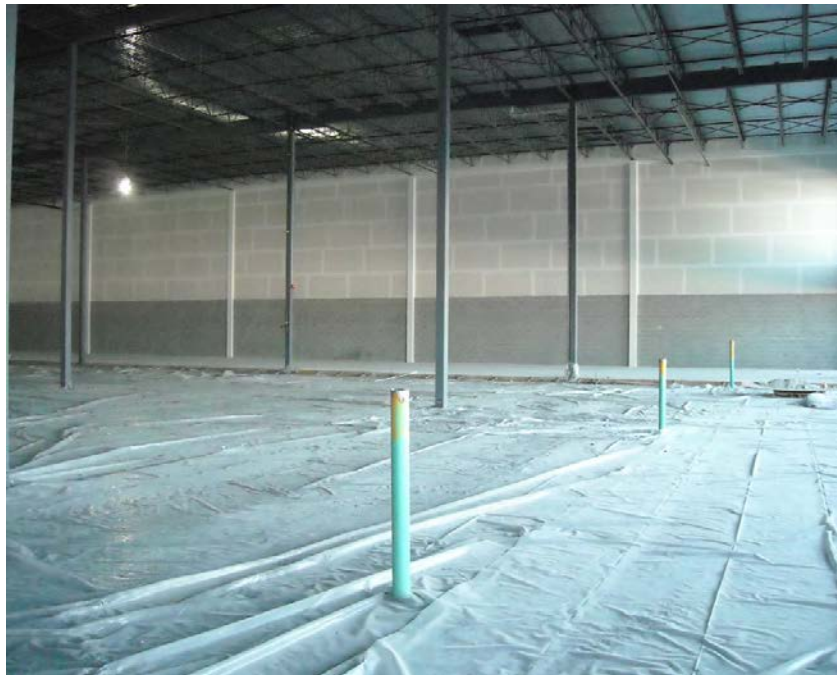
Figure 4: General view of a vacant and unfinished suite (3600 F.X. Tessier Street).
