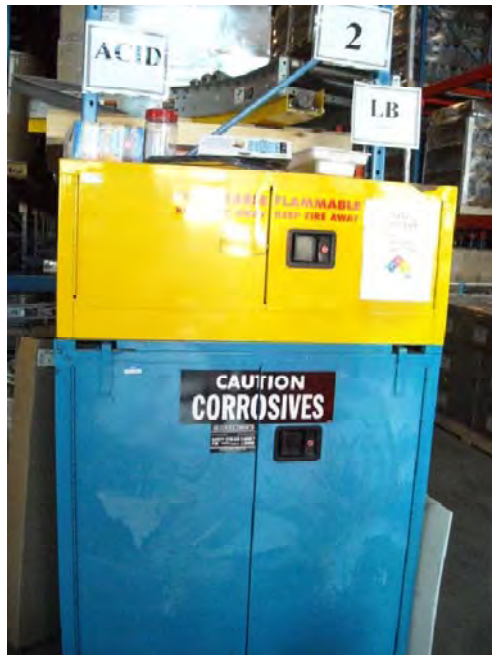
Figure 6: Partial view of flammable/corrosive products storage cabinet observed inside the suite occupied by Frenesius (3600 F.X. Tessier Street).
