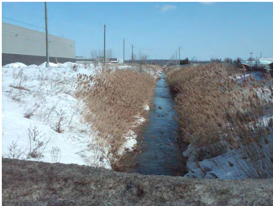
Figure 14: Partial view of the southern wall of the building located at 400 Marie-Curie Street and of the watercourse located southeast of the Site boundary.
