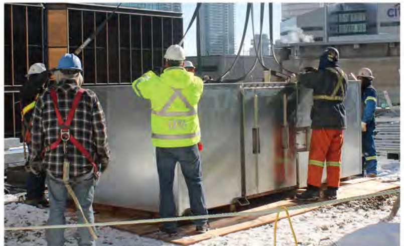
Safety Power has been able to achieve NO x reductions of up to 98% on a 2.5MW Tier 2 engine.
