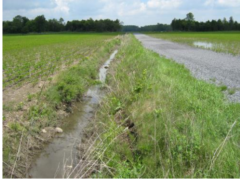
Ditch Adjacent to Runway South Threshold looking North
