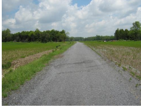
Southern Threshold Looking North along Runway Centreline
