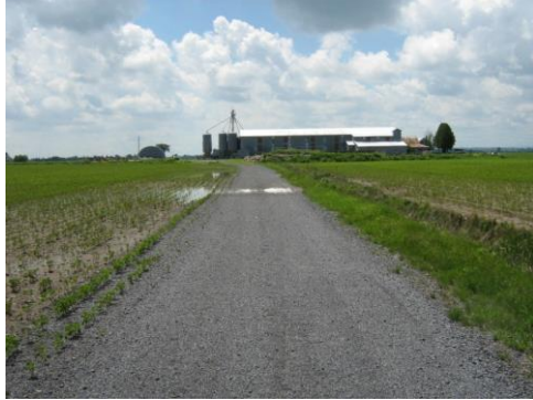
Southern Threshold Looking South along Approach
