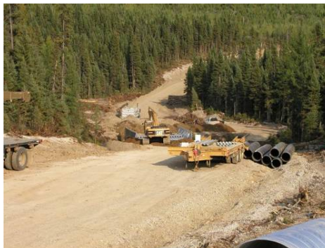
Construction de chemins forestiers
