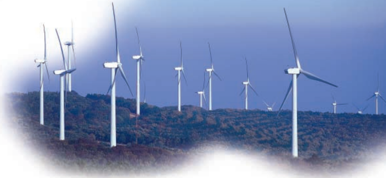
Escurillo, Spain 33 x 1.5sl, total capacity: 49.5 MW
