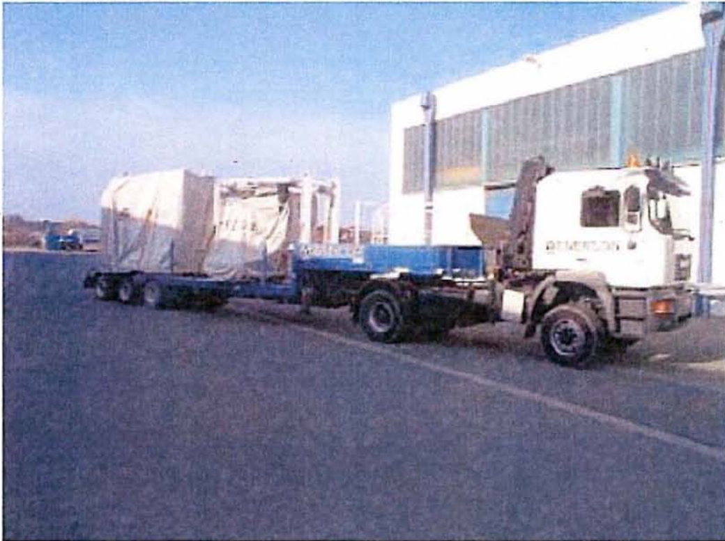
Figure 7 Transport of completed E-module to site
