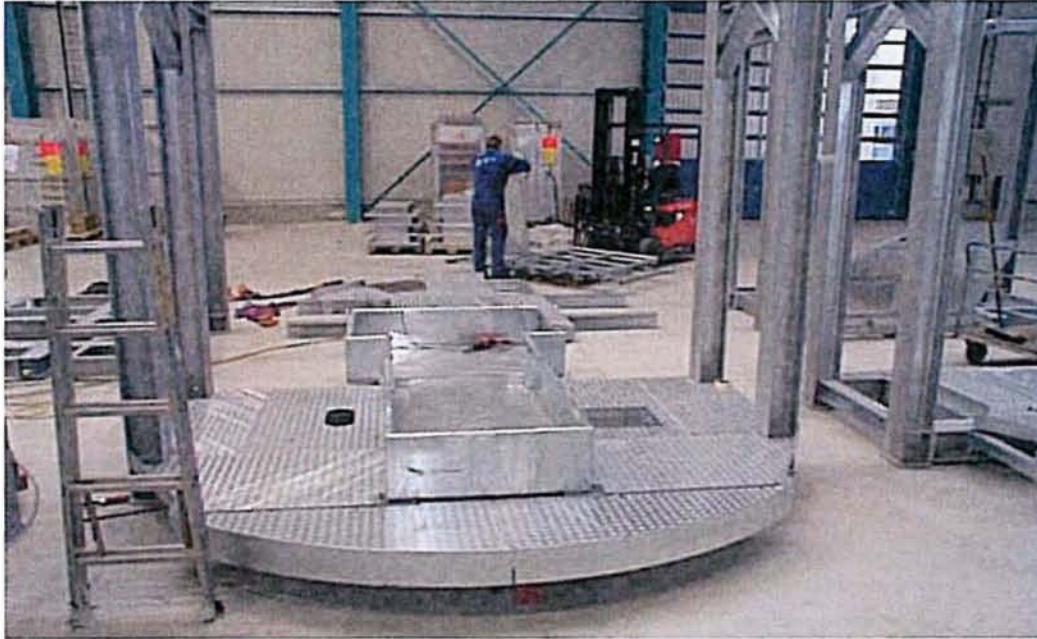
Figure 3 – Lower level ready to accept transformer and switchgear
