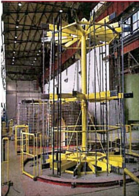
Figure – Assembly of the rebar
