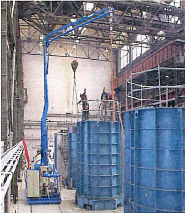
Figure – Concreting Process
