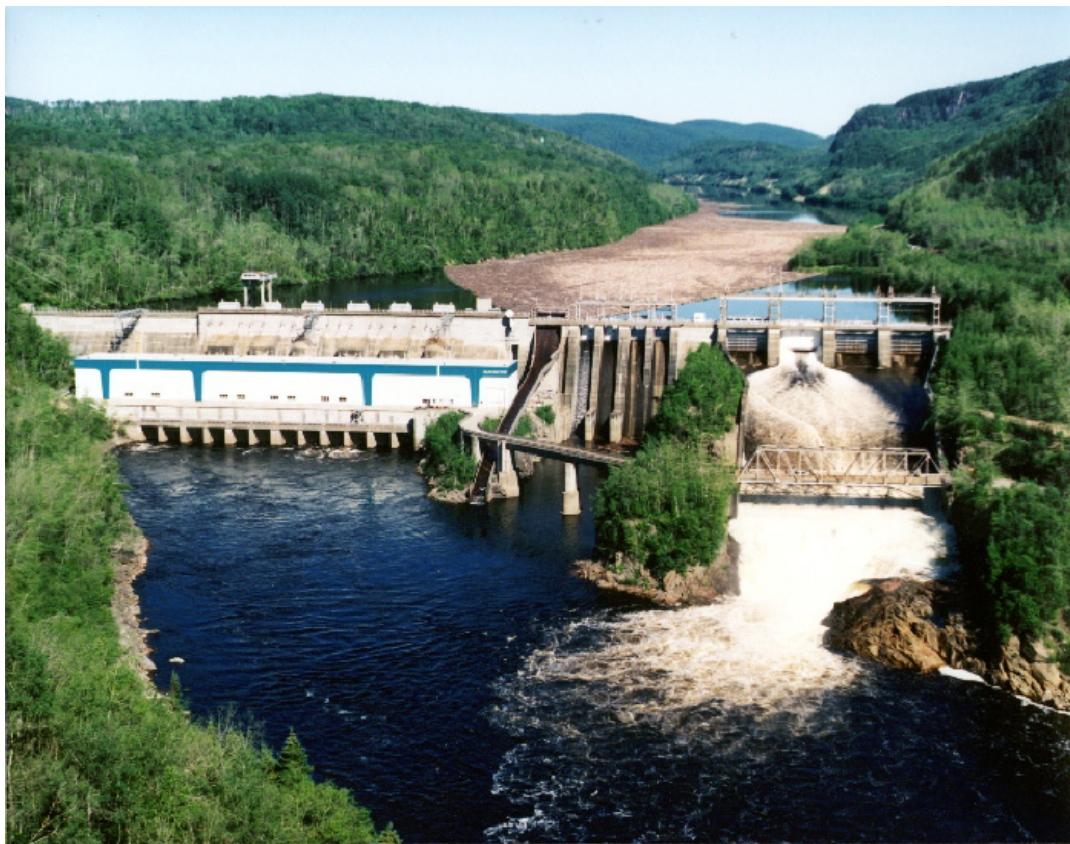
Figure 26 Photo de la centrale Beaumont
