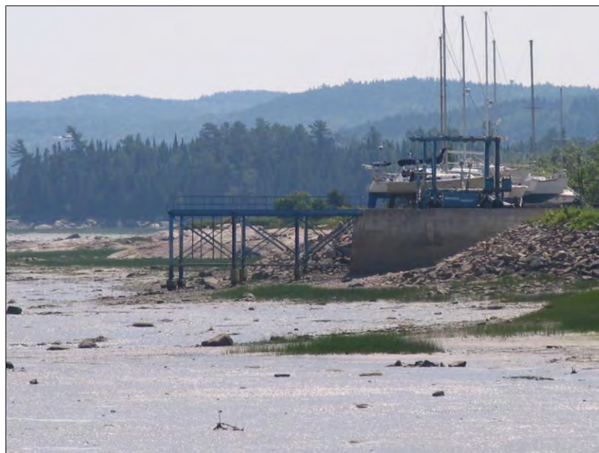
Figure 9. Occupation des infrastructures, Centre Nautique Saint-Martin.
