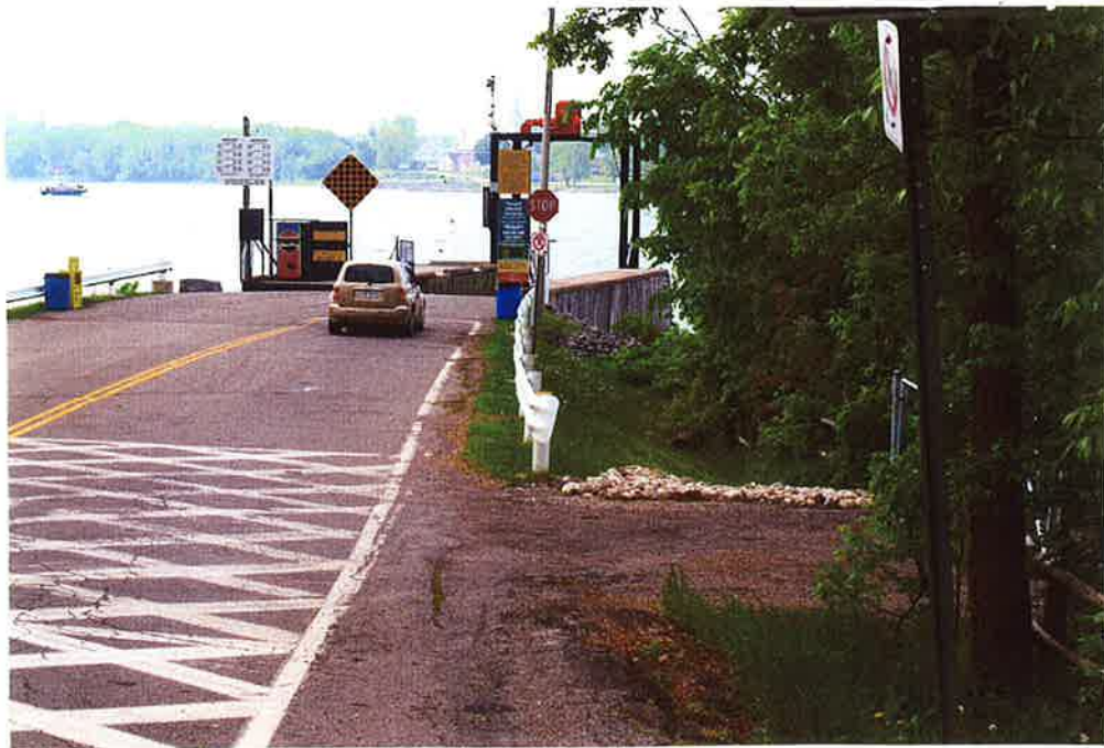
Figure 11B: Looking N at Mohrs Landing, downstream side
