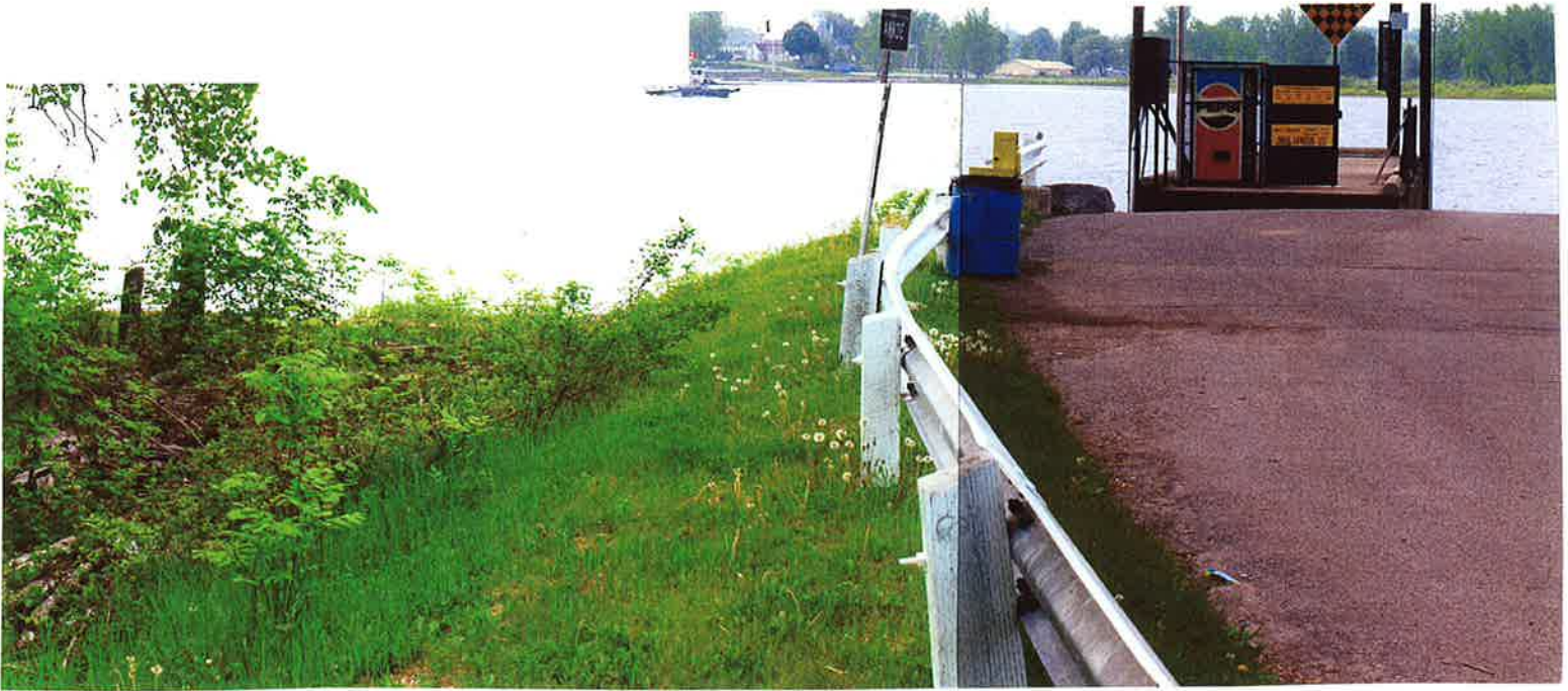
Figure 11A : Looking N at Mohrs Landing, upstream side
