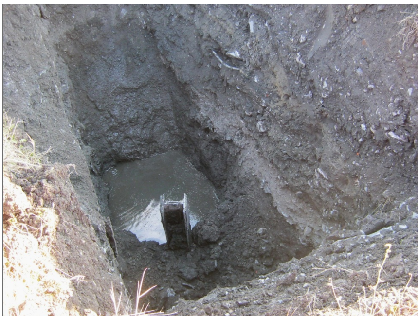
Photo 10: View of a metal support beam found at 3.5 m depth during the excavation of test pit TP-12-140.
