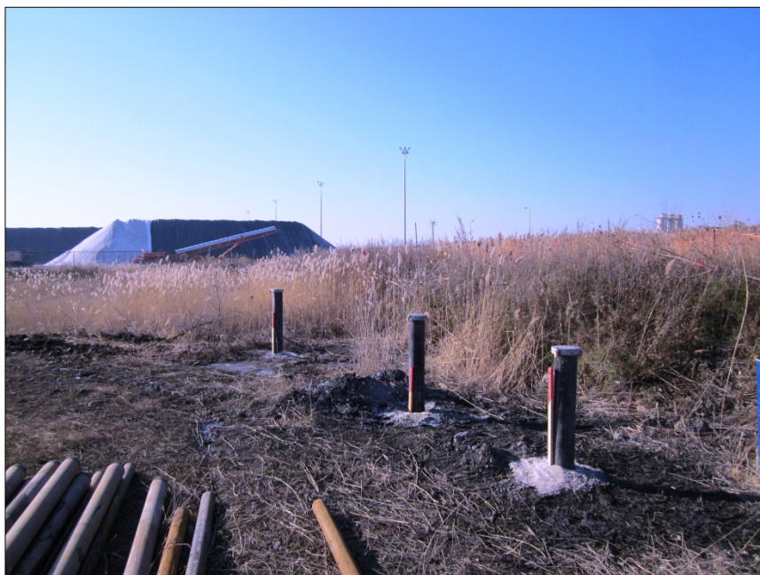
Photo 13: View of the completed cluster of monitoring wells MW-12-143, MWB-12-144, and MWC-12-145.
