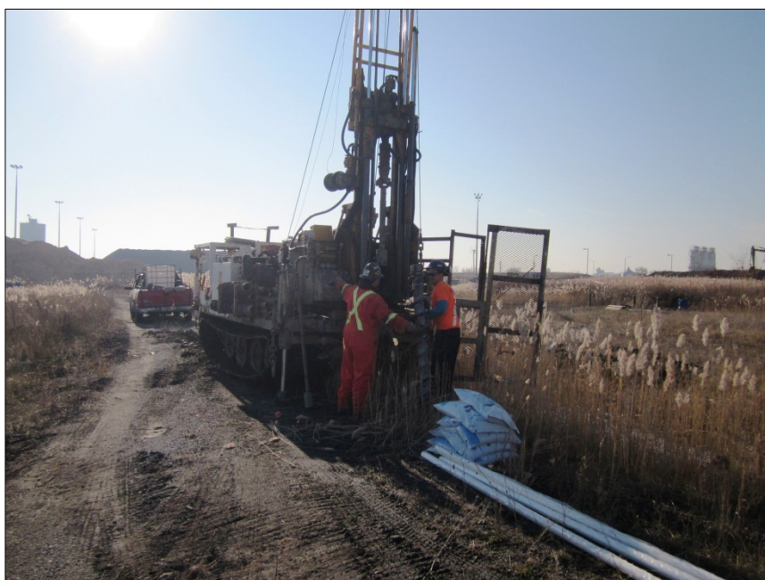
Photo 15: View of the monitoring well installation of MW-12-154.
