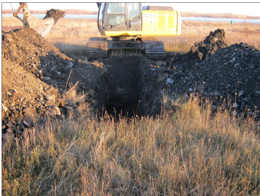
Photo 5: View of the excavation of test pit TP-12-132, located in the central portion of Site 1.
