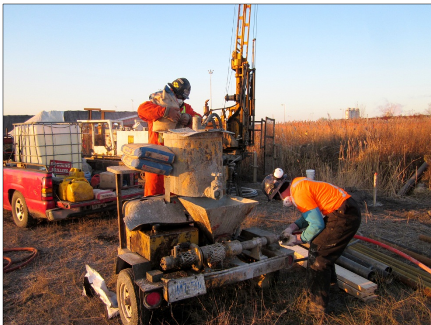
Photo 12: View of the preparation of the grout (cement-bentonite) for injection during the installation of bedrock monitoring well MW-12-145.
