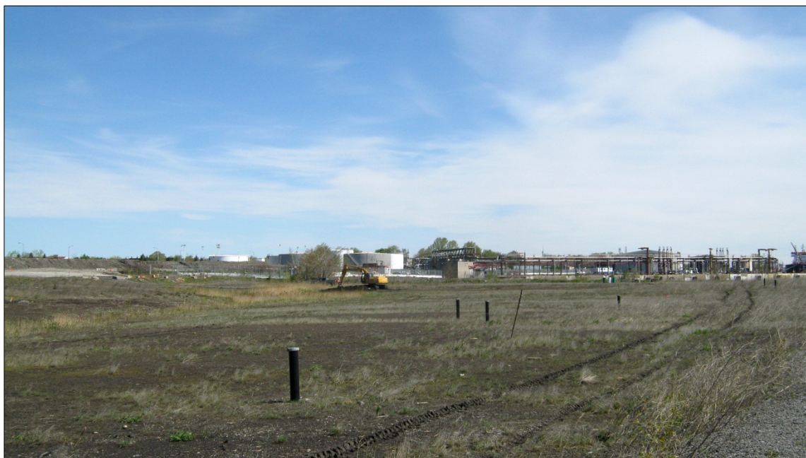
Photo 3: View of the excavation of a test pit in May 2012, looking towards the north. Also note the previous existing wells in the forefront.
