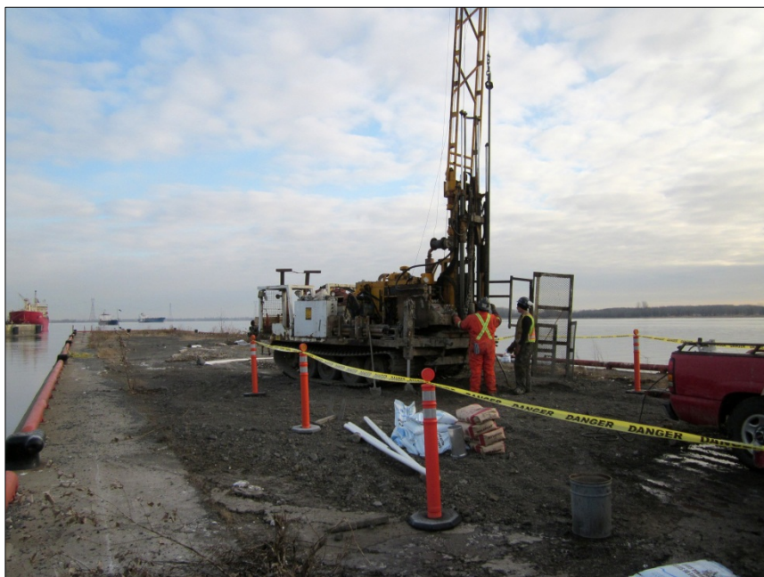
Photo 19: View of the drilling activities at MW-12-181, located along the pier, in the northern portion of Site 1.
