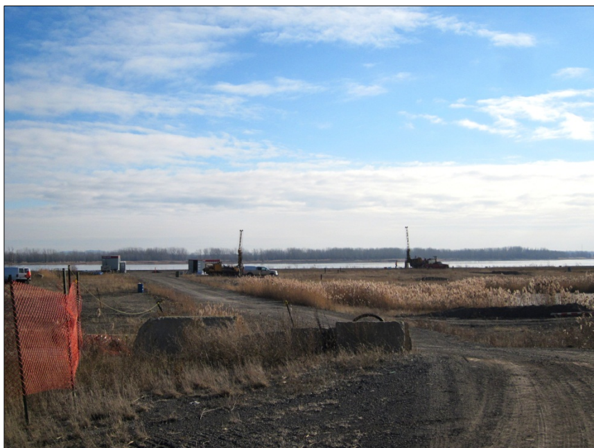
Photo 2: View of the drilling activities of the two drill rigs present on Site 1, in the northeastern corner of the property.
