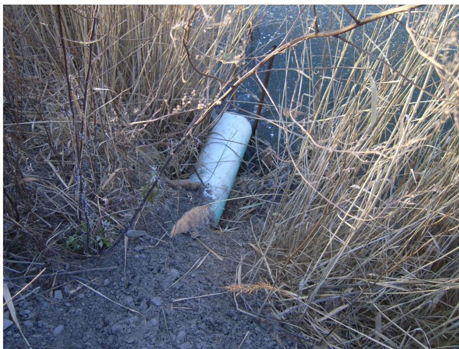
Figure 8: Drainage pipe observed on the western side of the 50 m by 15 m drainage pond, inferred to connect with the adjacent drainage trench.
