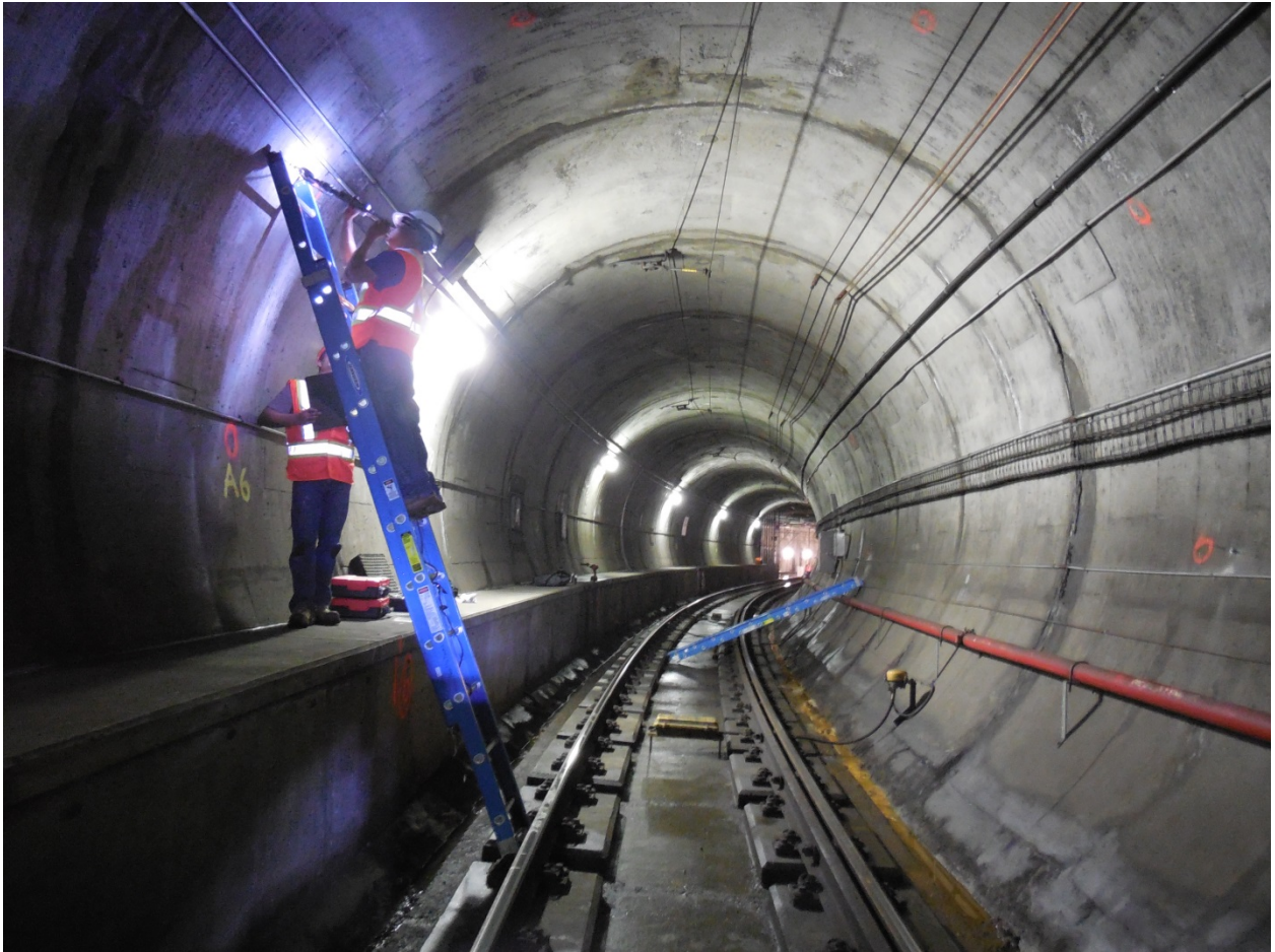
Figure 5-31 : Tunnel Mayfair - Edmonton LRT
