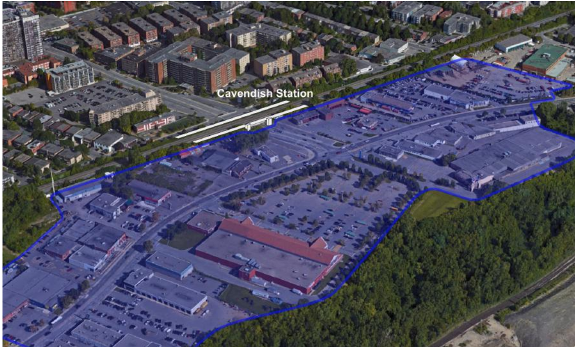
Proposed Cavendish station with potential TOD development area. The area represents about 170,00 m 2 , 41.93 acres, 0.170km 2 (source: Google, modified by Anton Dubrau)
