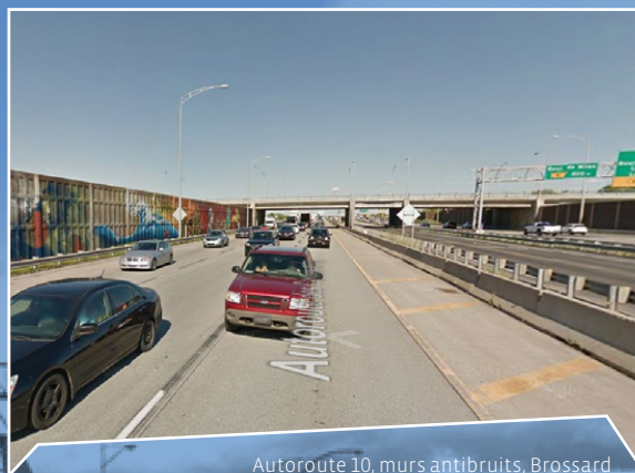
Autoroute 10, murs antibruits, Brossard
