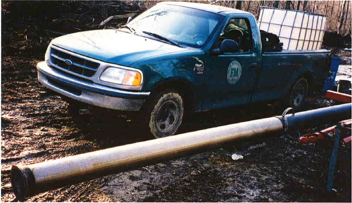
8. Crépine du puits de pompage PP-03-01 / Screen of pumping well PP-03-01
