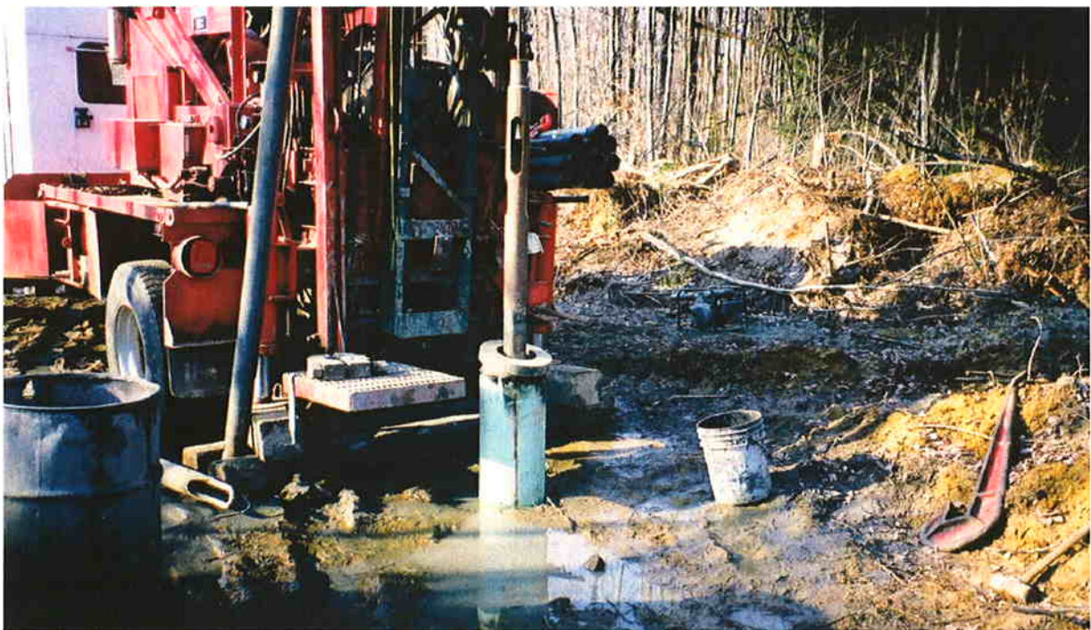
7. Forage du puits de pompage PP-03-01 / Drilling of pumping well PP-03-01
