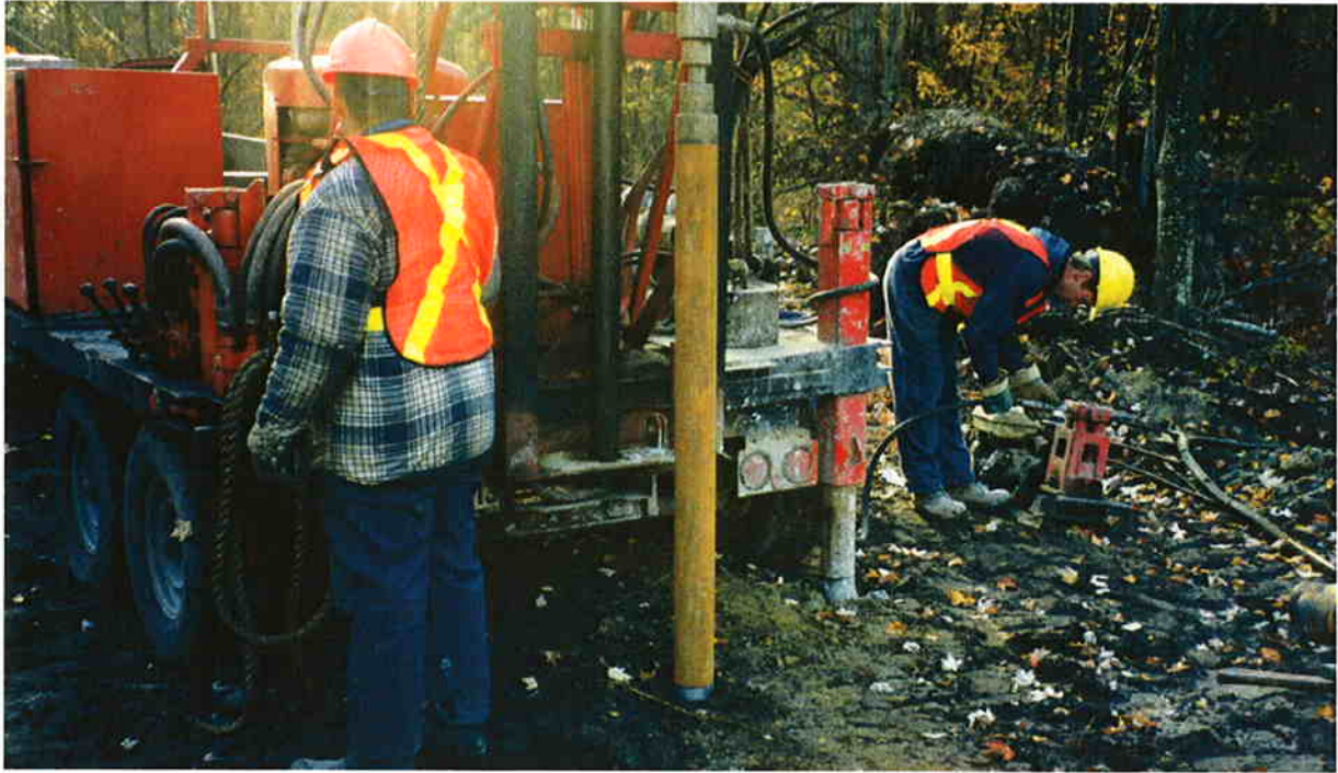
1. Forage du puits PO-03-01A / Drilling of well PO-03-01A
