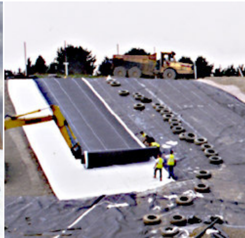
Figure 3 - Covering of a GCL by a Geomembrane thereby Forming a Composite liner, i.e., a GM/GCL Composite
