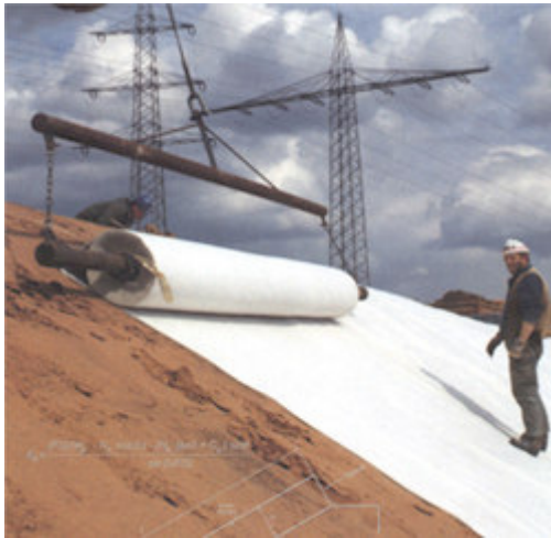
Figure 2 - A GCL Being placed on a Side Slope
