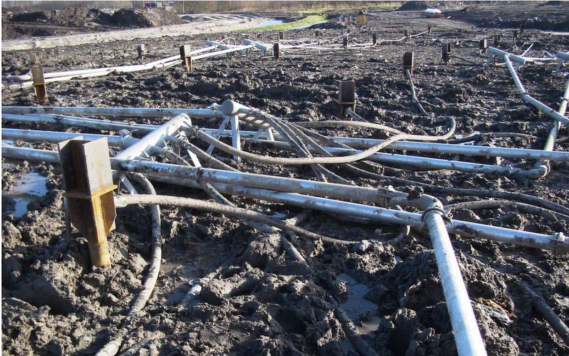
Figure 5. The aeration of waste
