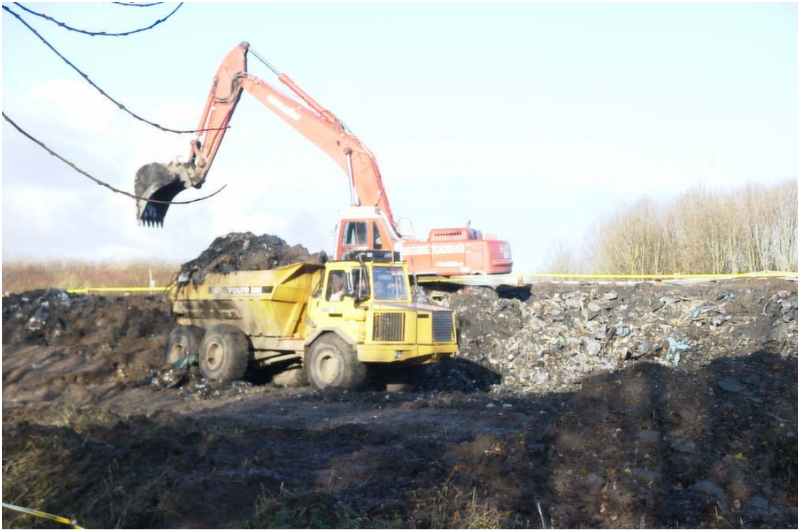
Figure 1. Excavation of non aerated waste at Zeeasterweg landfill
