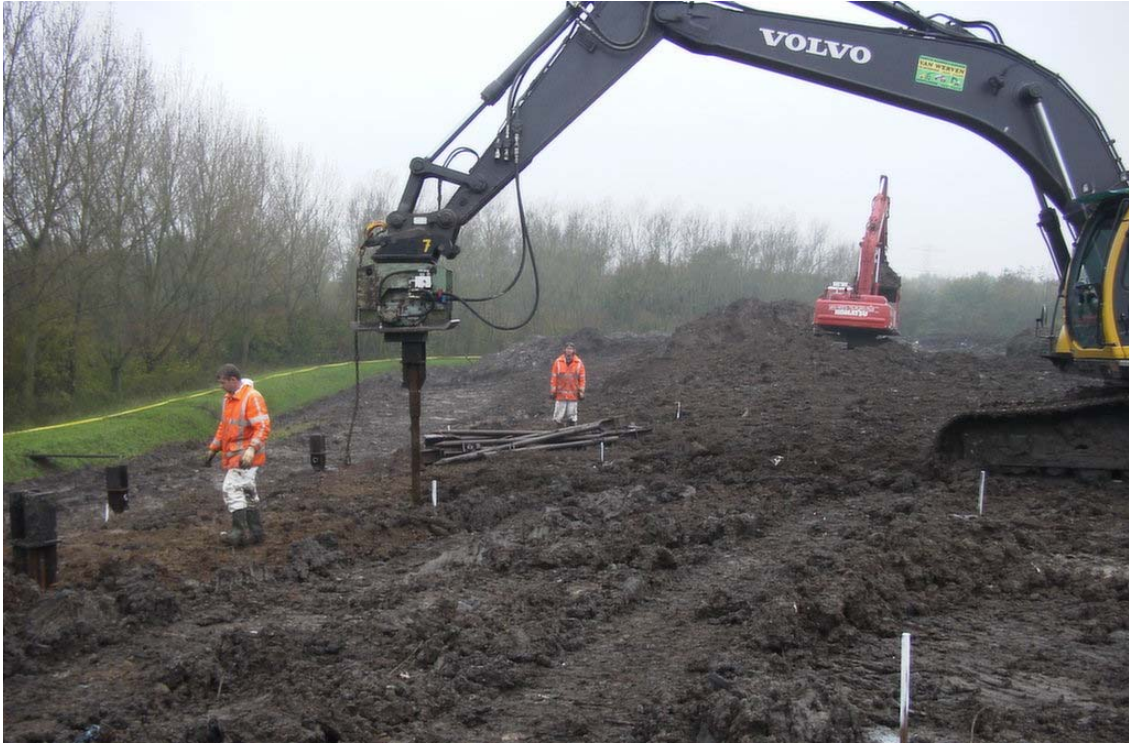
Figure 2. Installation of the aeration system
