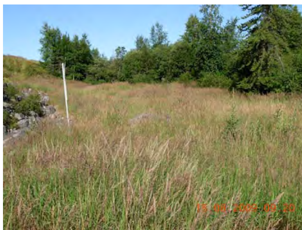
Figure 8: Downstream toe area after vegetation control
