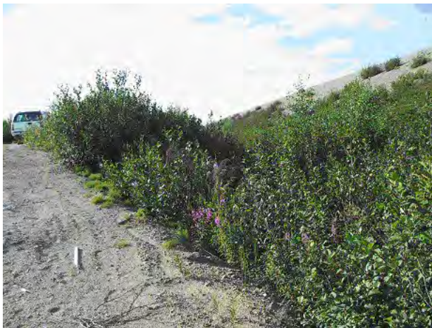
Figure 14: Downstream slope and toe area
