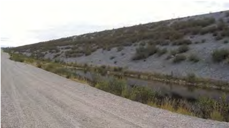
Figure 16: Downstream slope of a 30-year old embankment
