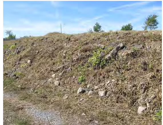
Figure 3: Slope after vegetation control
