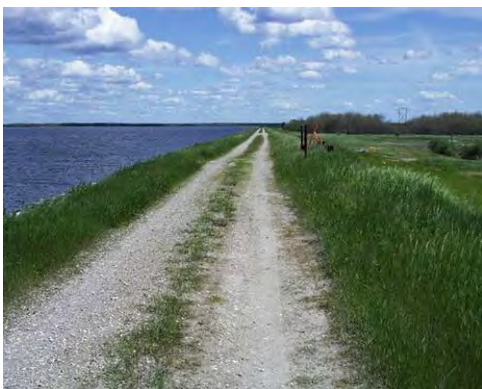
Figure 19: Crest of the embankment
