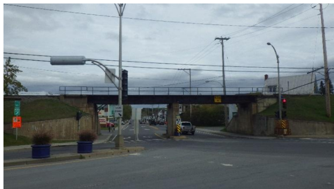
Figure 2-E P.M. 116.96 – Viaduc ferroviaire (BTPG)
