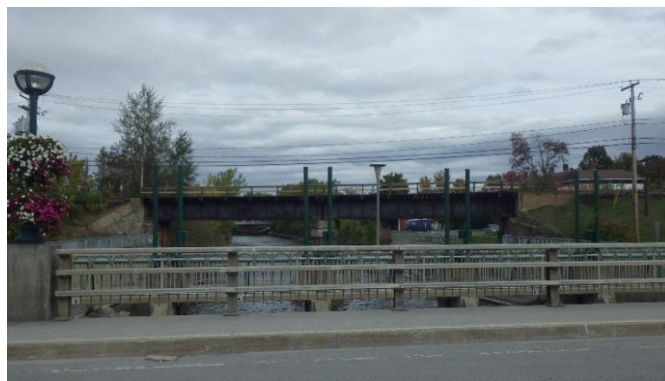
Figure 2-F P.M. 117.02 – Pont ferroviaire (DPG)
