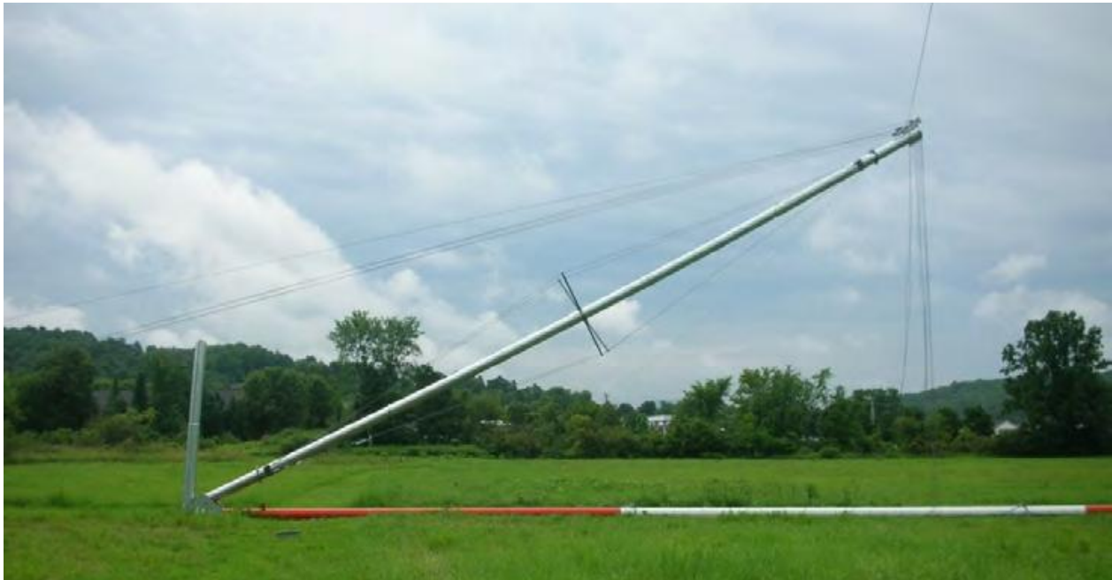
Figure 3. Érection du mât de levage (ginpole)
