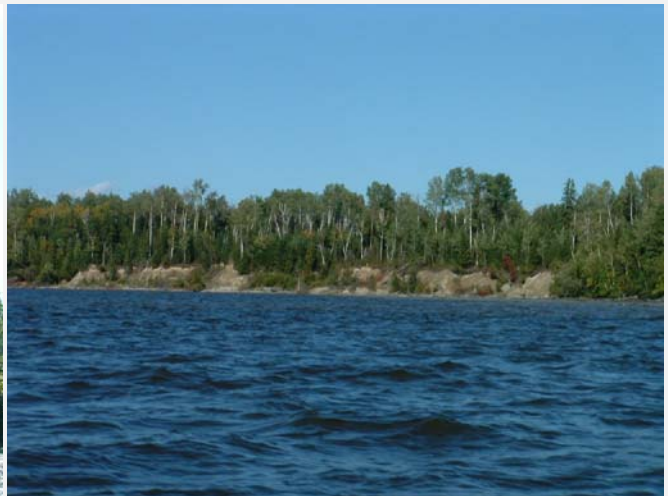
East bank of the Des Quinze lake eroded by waves
