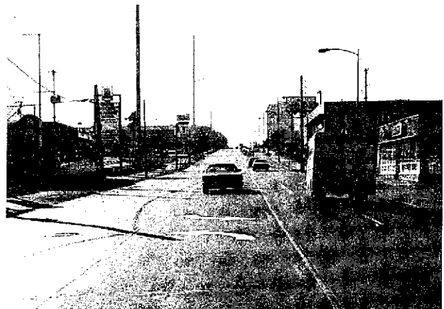
Figure 7. Five-lane divided highway with center two-way left-turn lane.
