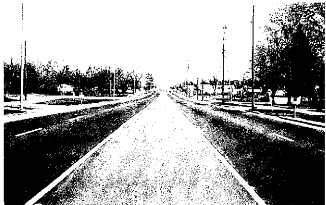
Figure 8. Five-lane divided highway with center two-way left-turn lane.
