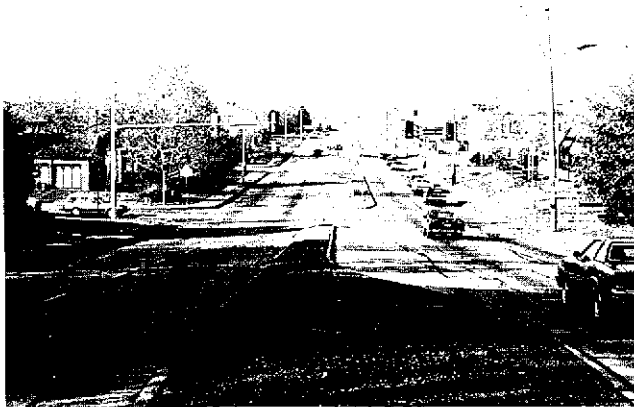
Figure 9. Five-lane divided highway with continuous alternating left-turn lane and raised median.
