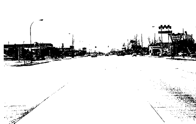
Figure 12. Seven-lane divided highway with center two-way left-turn lane.
