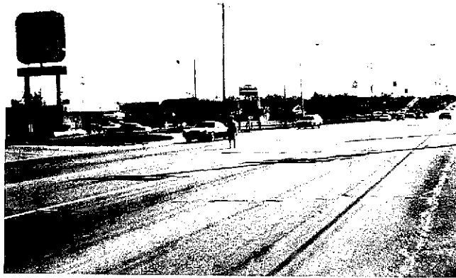
Figure 15. Problems encountered by pedestrian crossing a five-lane divided highway with TWLTL.
