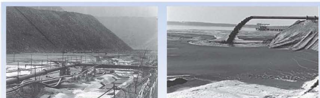
Helmsdorf tailings disposal area during operations: tailings were deposited in a shallow valley adjacent to the processing plant, contained by two dams constructed of waste rock. No bottom liner for groundwater protection was installed prior to operation and little consideration was given to the potential impacts from leakage or a dam failure on communities located downstream of the impoundment.
