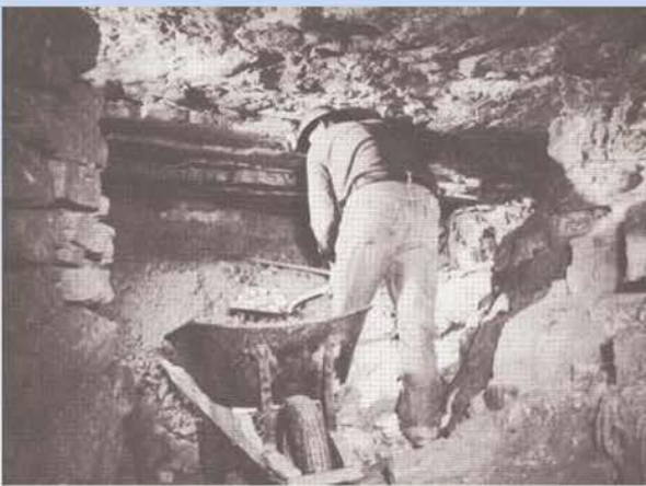
Hand loading ore onto a wheelbarrow in a small mine on the Colorado Plateau in the mid-1950s. In early operations, miners were not properly trained and hazards were not well-understood. As a result, injury and fatality rates were high.
