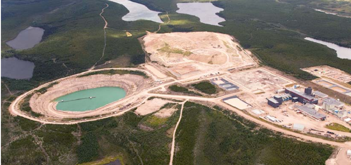
Figure A3: Aerial view of the JEB site, north end of the McClean Lake Operation
