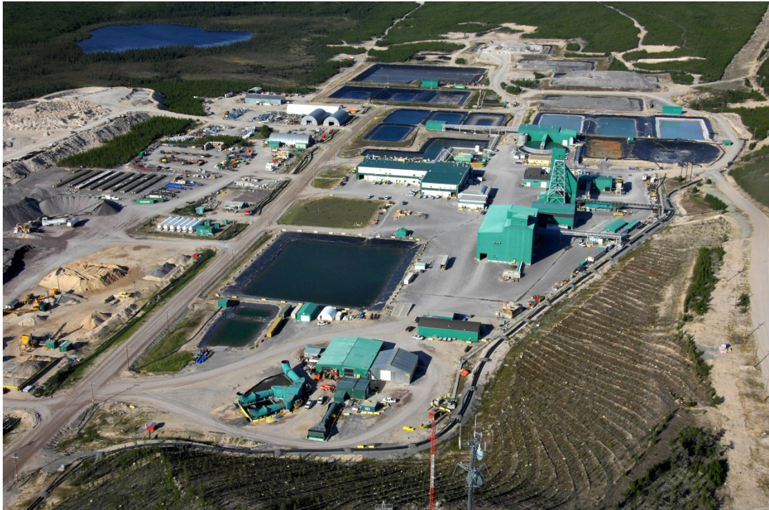
Figure A10: Aerial view of the McArthur River Operation
