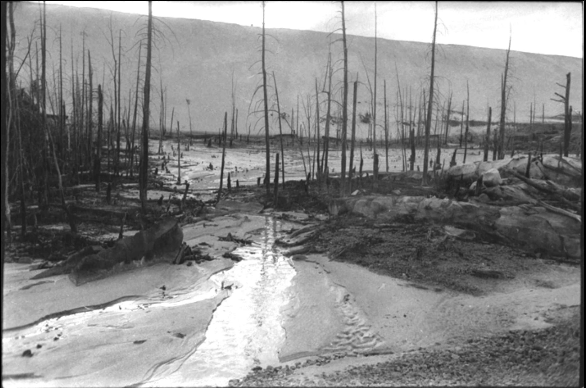
This 10-metre high wall is part of a deposit of 70 million tonnes of U tailings in Elliot Lake area.
