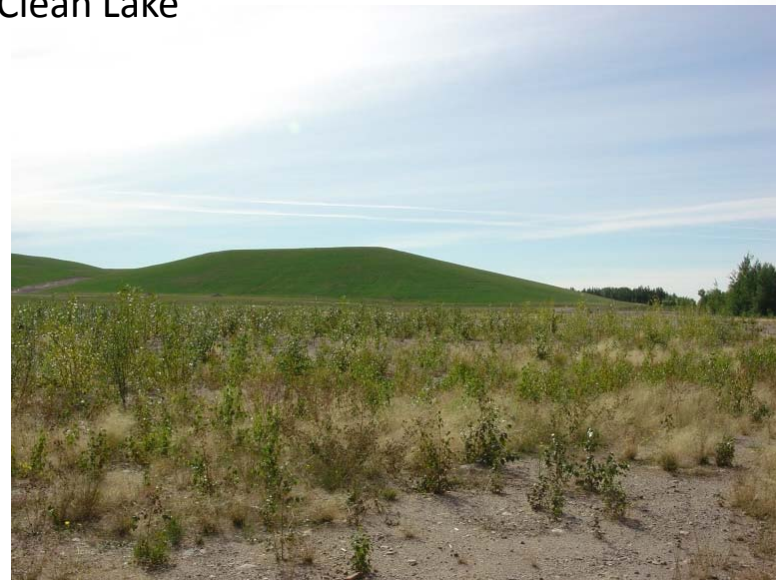
Surface management with cover designed to limit water infiltration and exposure to oxygen – Example of Cluff Lake
