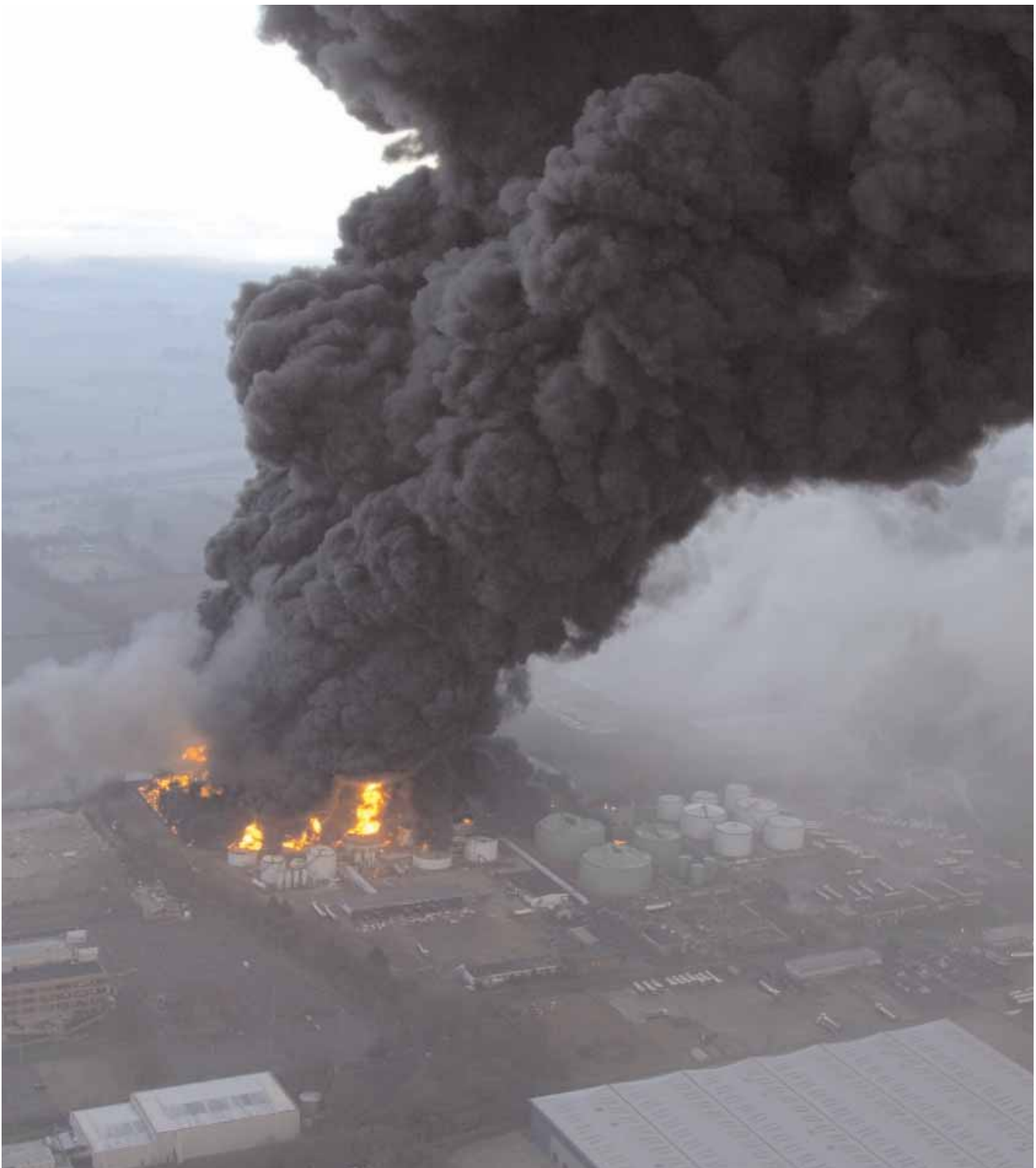
Figure 3 The smoke plume rising and spreading above the Buncefield site.
