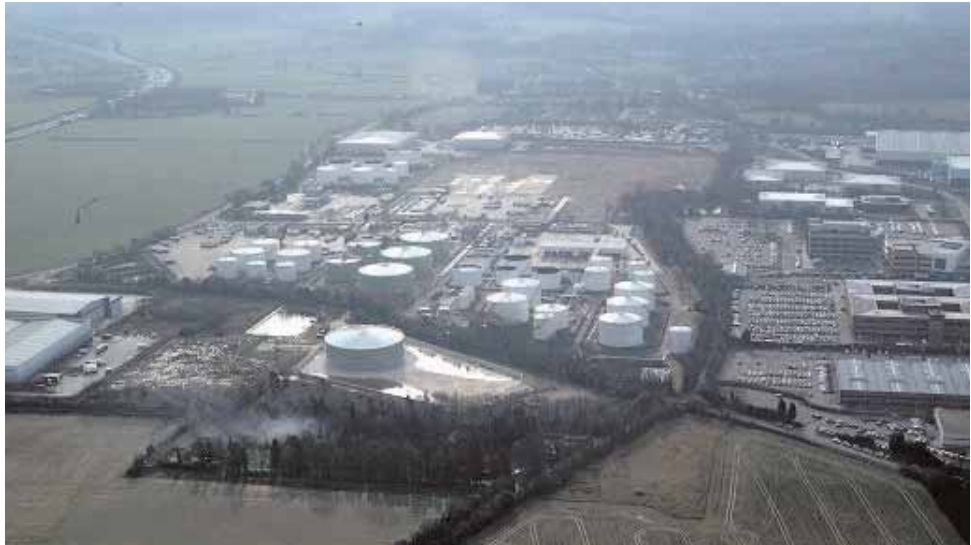
Figure 7 The area prior to incident
