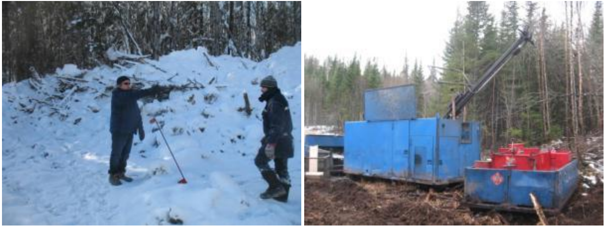
Figure 5.5.1 General Drilling Conditions at Paul in February and November 2012
