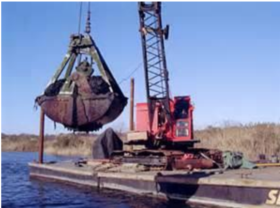
Figure 10: Clam shell excavation in water
