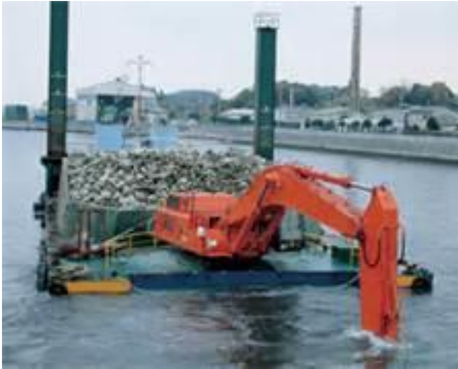
Figure 9: Backhoe excavations in water placing spoils on barge
