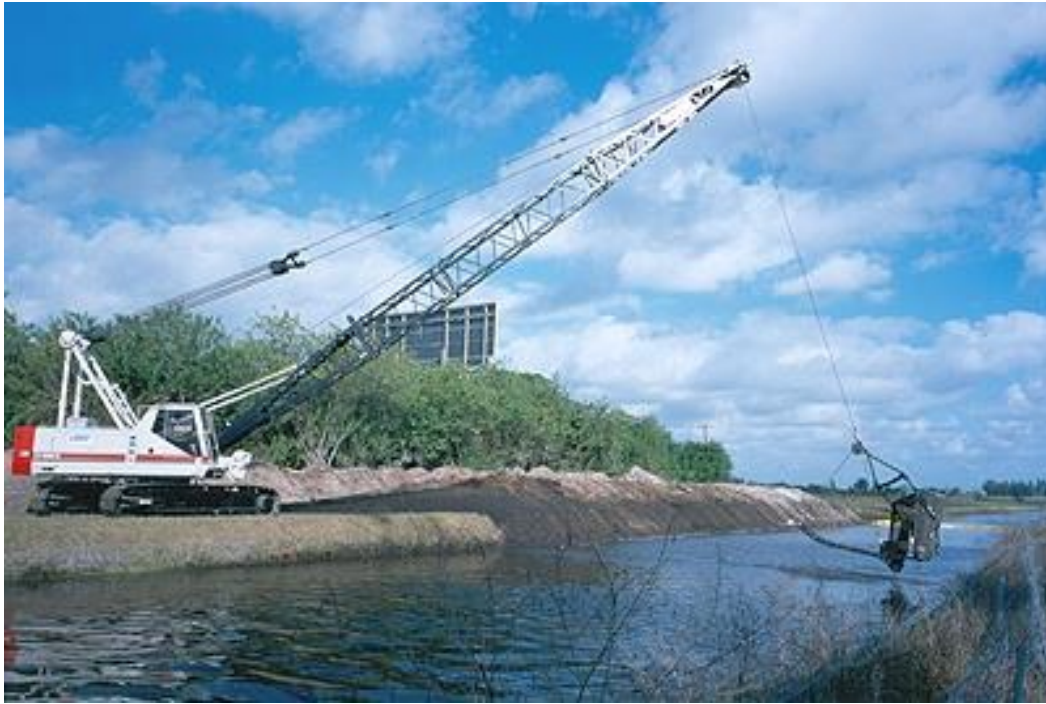
Figure 11: Dragline excavations in water
