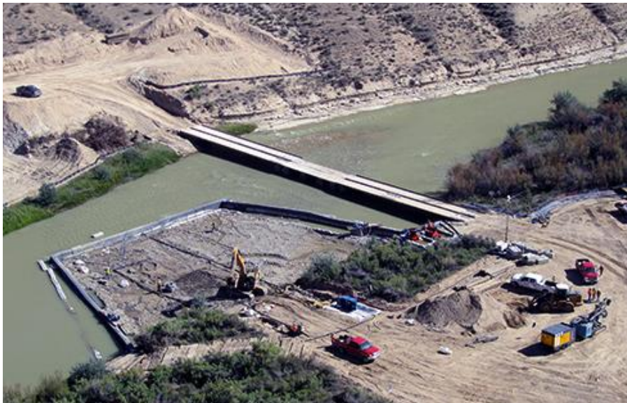
Figure 17: Typical dry open cut trench crossing
