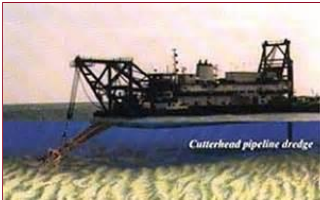
Figure 14: Photo of a dredge illustrating the excavation of a trench in the water
