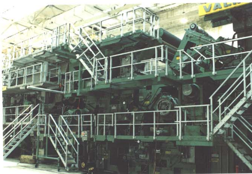
Corner Brook Pulp & Paper Ltd, Corner Brook, Terre-Neuve
