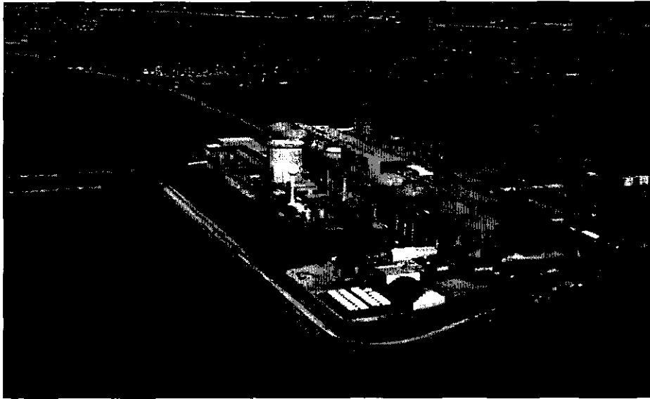
Pickering Nuclear Generating Station (see paragraph 27.12).
