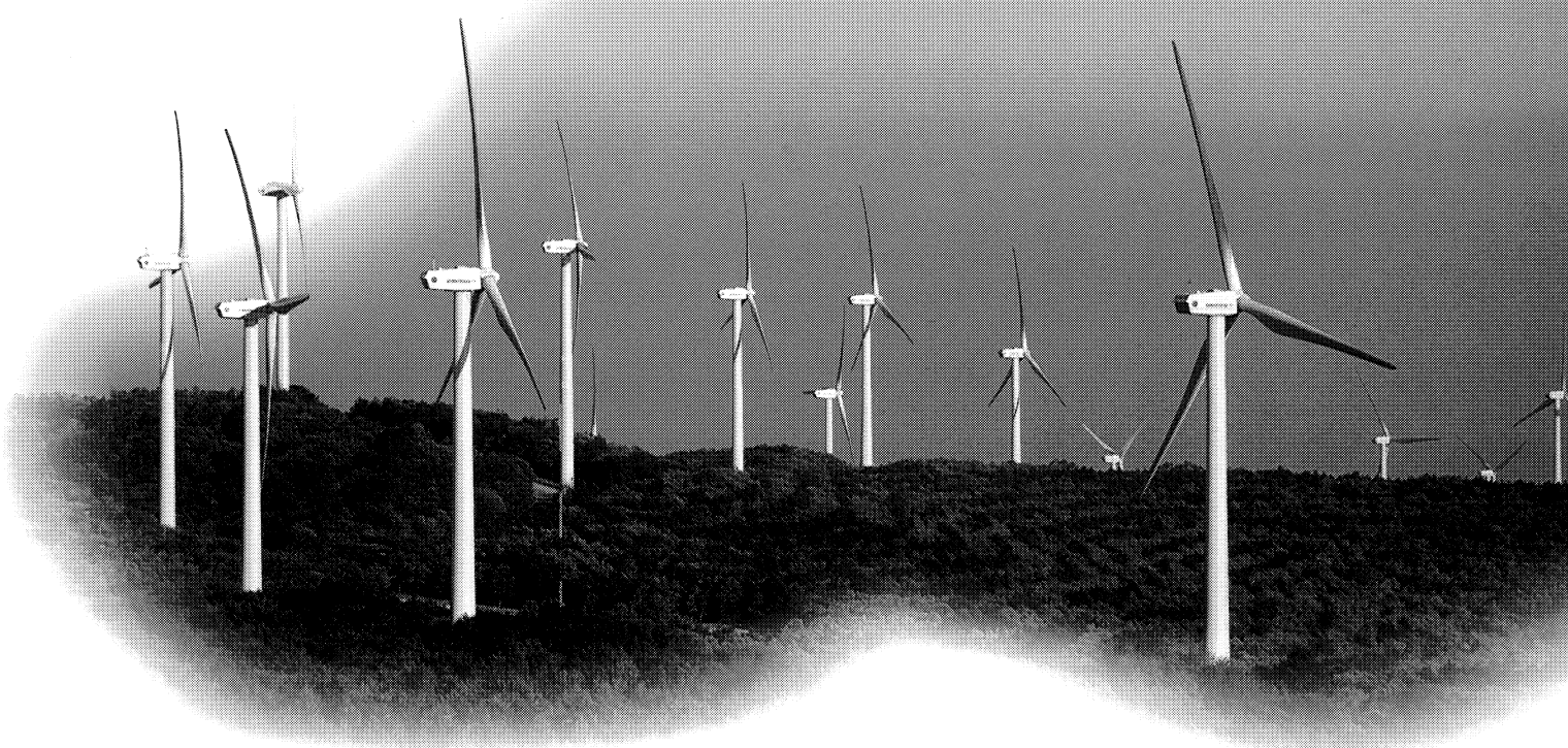
Escurillo, Spain 33 x 1.5sl, total capacity: 49.5 MW
