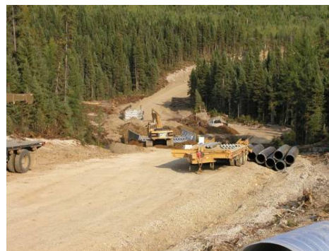
Construction de chemins forestiers
