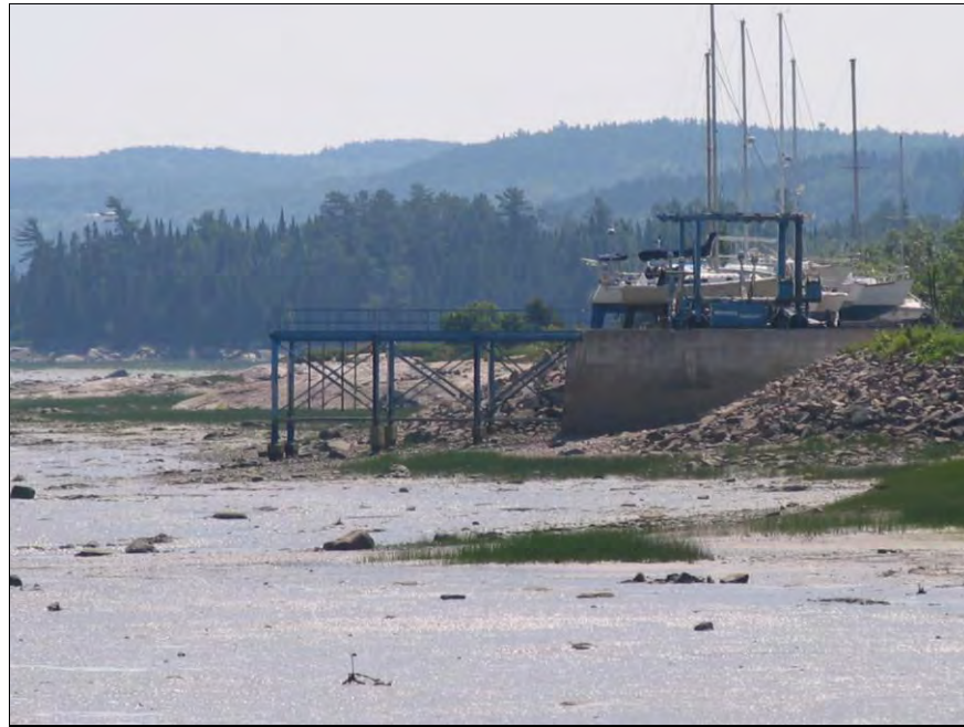
Figure 9. Occupation des infrastructures, Centre Nautique Saint-Martin.
