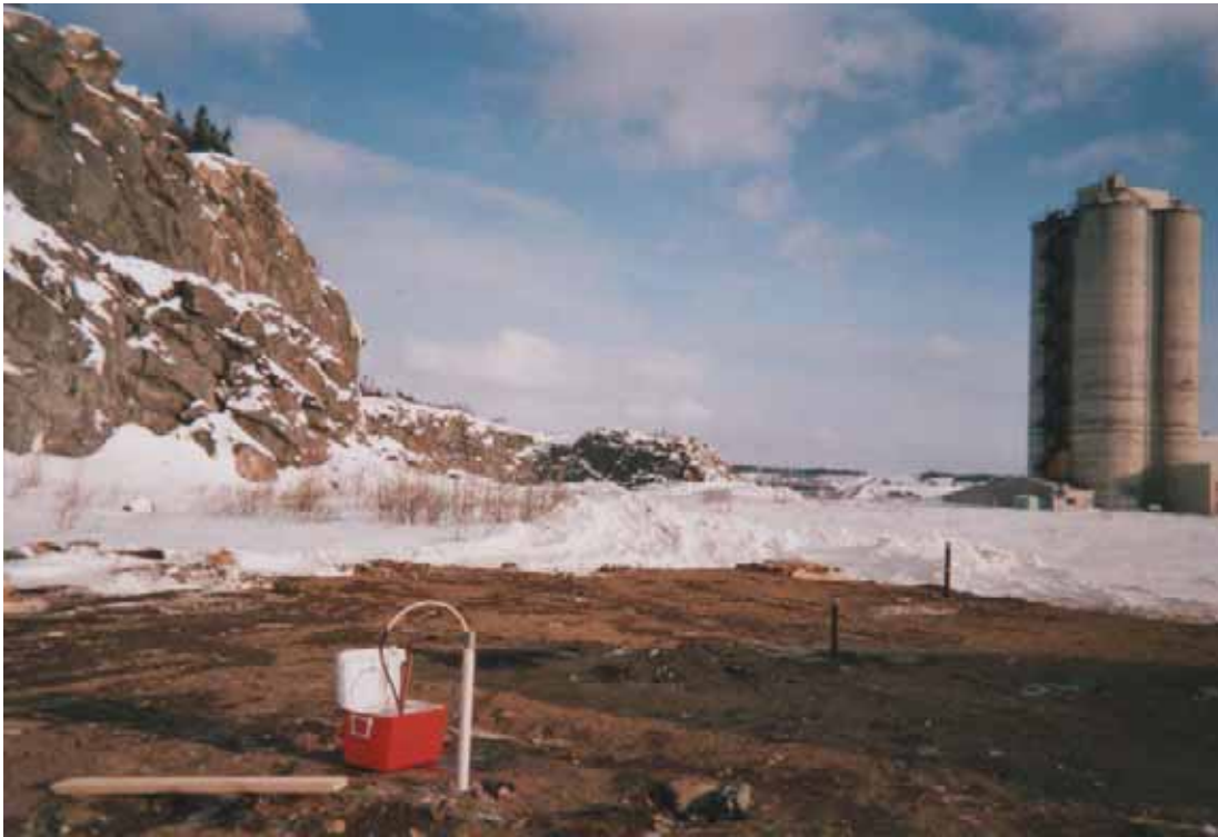
Photo 8. View of three in-line boreholes (8m apart) used for conducting the cross-hole seismic survey in the footprint of tank T-101. Borehole BH-7 (HQ-75mm) was drilled to a depth of 30m and showed the rock to be solid (strong) below the initial 0.5 metres of blast rock on the surface and 2m of fractured, blast affected rock.
