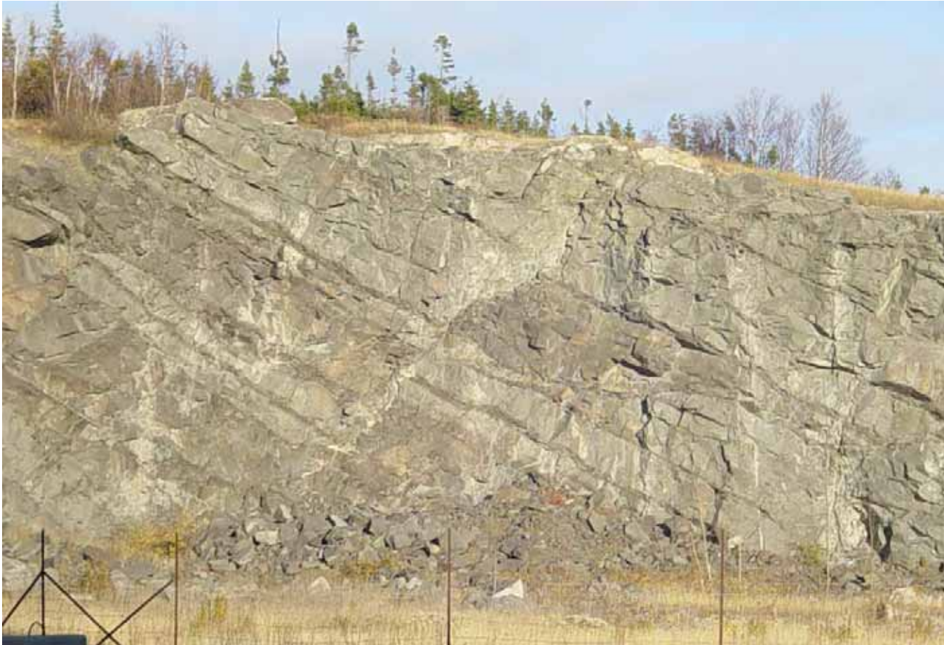
Photo 13. Clearly defined fault, with approximately 2.5m of vertical offset, south of future tank site (south west of cement silos). No indication of recent movement on fault plane. Fault plane passes approximately 200m east of and slopes away from future tanks and does not effect the tank foundations.
