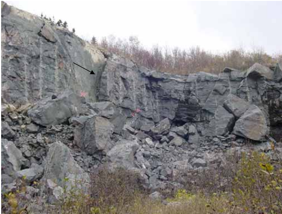
Photo 7. Area view of a sub-vertical fracture (photo looking south-east). The fracture plane separating the two massive sandstone beds continues through tank T-101.
