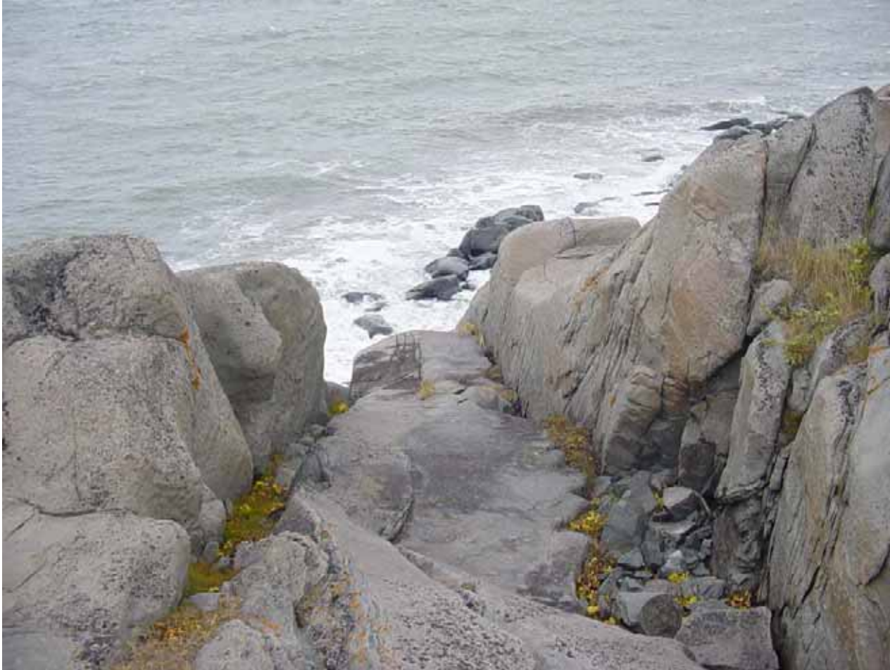
Photo 20. Near vertical series of joint planes orientated NE-SW. Note vertical grooves in northern rock face (right). Features are likely caused by wave erosion but the underground extension of feature should be observed during future works or excavations to confirm that it does not effect the foundation for tank 2-future.
