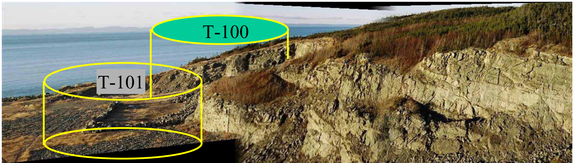
Photo 2. View looking across tank T-101 and T-100 sites towards the St. Lawrence (North).
