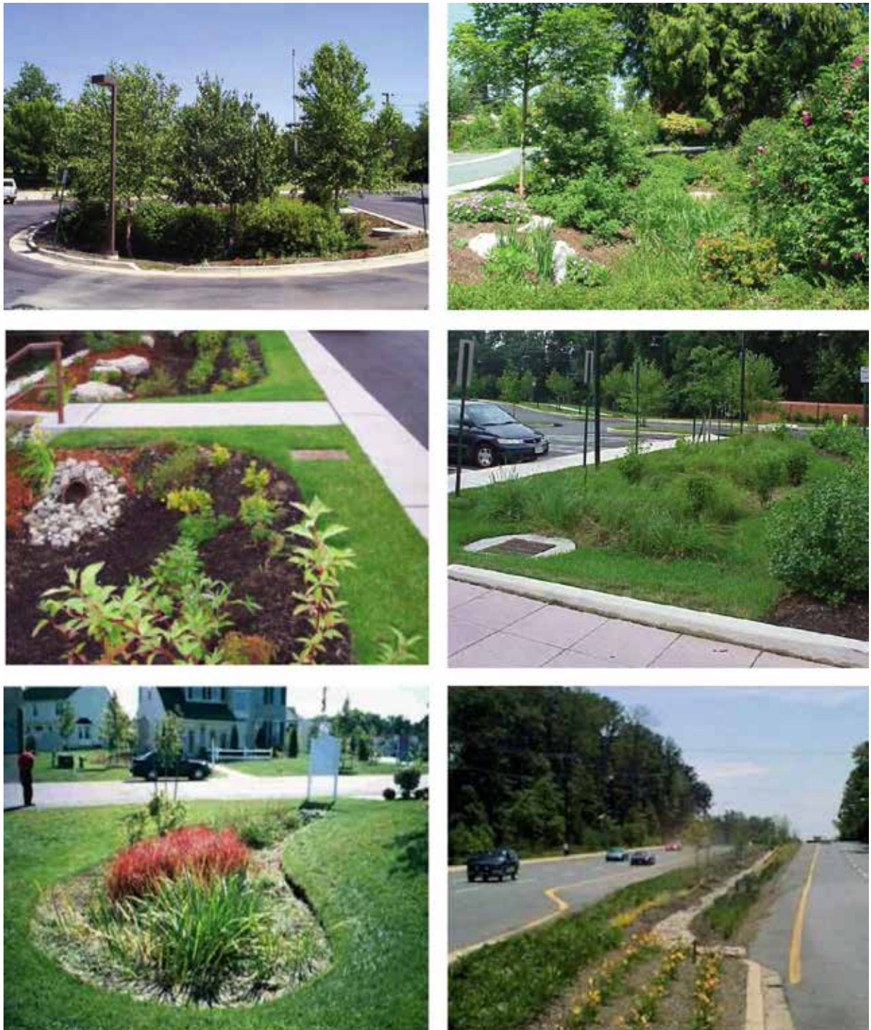
Figure 11.28 Applications diverses de la biorétention.
