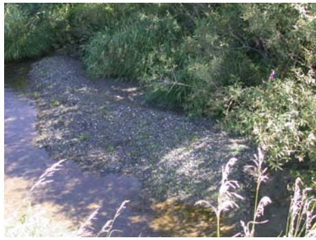
Pt 25: Accumulation de gravier
